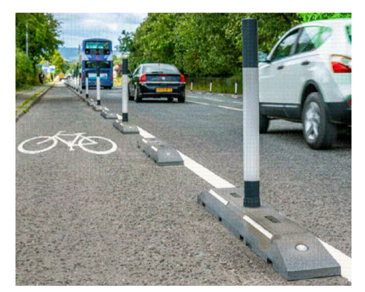
Fig 1. ROSEHILL NARROW CYCLE LANE DEFENDER UNITS - TO PROVIDE TRAFFIC SEGREGATION. PRODUCT 2.0m IN LENGTH & ARE BOLTED INTO CARRIAGEWAY WITH 5m GAP. NOTE CONTINUOUS WHITE LINING 1.8m OFFSET FROM KERB ON ROAD SIDE OF DEFENDER.
