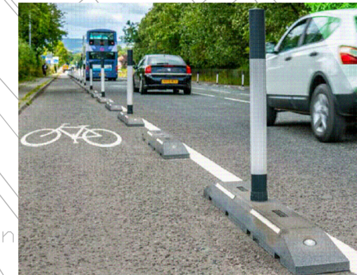
Fig 1. ROSEHILL NARROW CYCLE LANE DEFENDER UNITS - TO PROVIDE TRAFFIC SEGREGATION. PRODUCT 2.0m IN LENGTH & ARE BOLTED INTO CARRIAGEWAY WITH 5m GAP. NOTE DEFENDER TO BE POSITIONED OFFSET 1.5m FROM KERB WITH CONTINUOUS WHITE LINING AT 1.8m OFFSET FROM KERB.
