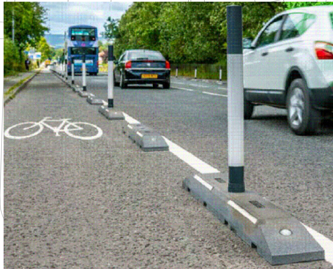
FIG 1. ROSEHILL NARROW CYCLE LANE DEFENDER UNITS - TO PROVIDE TRAFFIC SEGREGATION. PRODUCT 2.0M IN LENGTH & ARE BOLTED INTO CARRIAGEWAY WITH 5M GAP. NOTE CONTINUOUS WHITE LINING ON ROAD SIDE OF DEFENDER.
