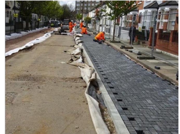
Figure 52. Retro fitting permeable paving, Mendora Road, Fulham | Atkins
