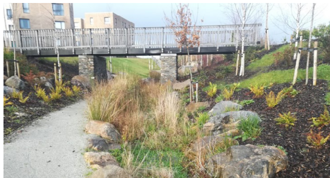
Figure 2. Swales at Countesswells, Aberdeen | SNH
