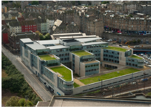
A | Green Roofs
