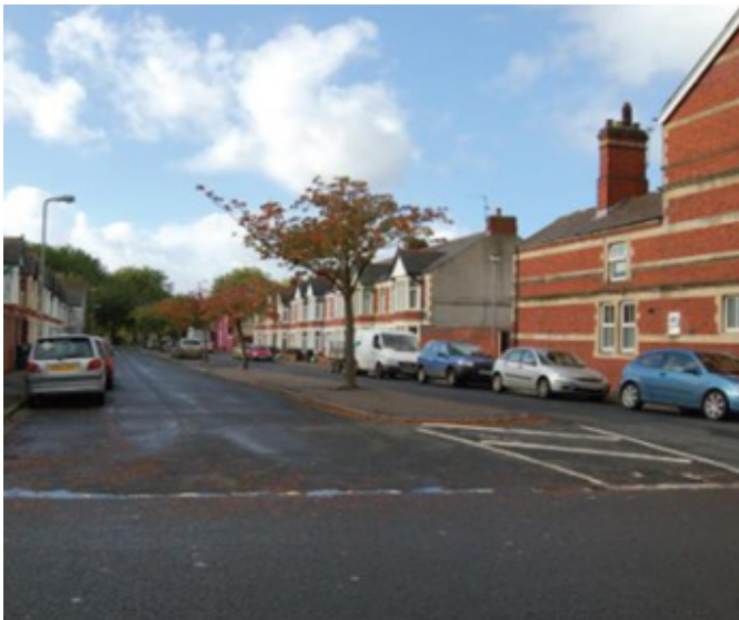
Figure 78. Grangetown before SuDS scheme | Atkins
