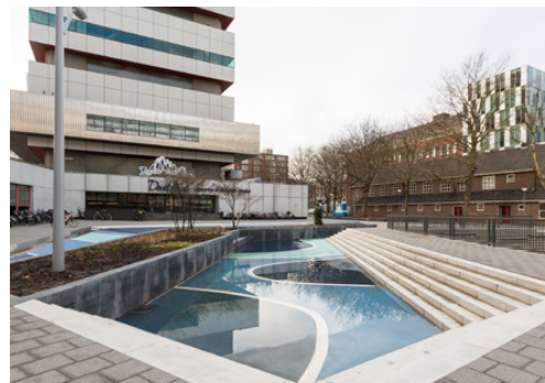
J | Hard Detention Basin
