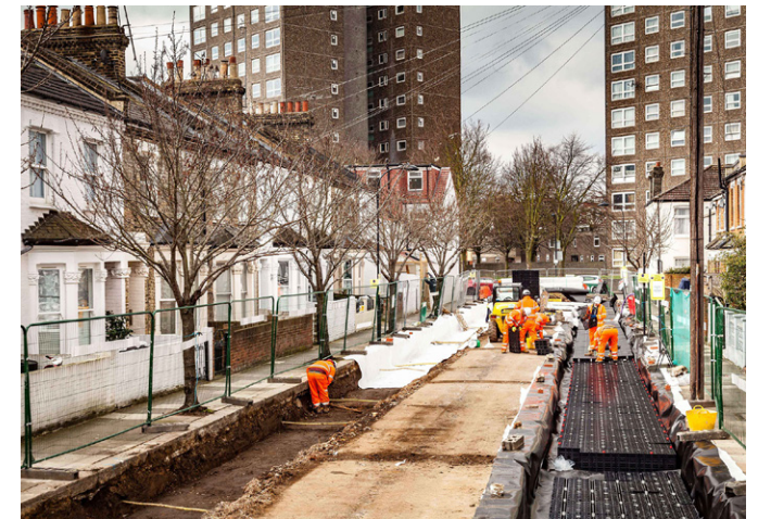
Figure 61. Geocellular systems under construction, Mendora Road, Fulham | Atkins
