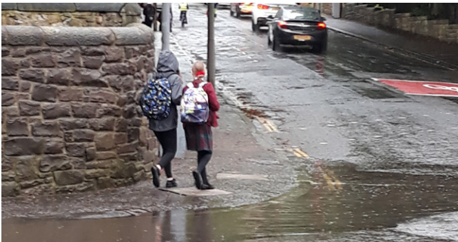
Figure 21. Road Gullies overwhelmed by rain, Polworth Edinburgh June 2019 | Atkins
