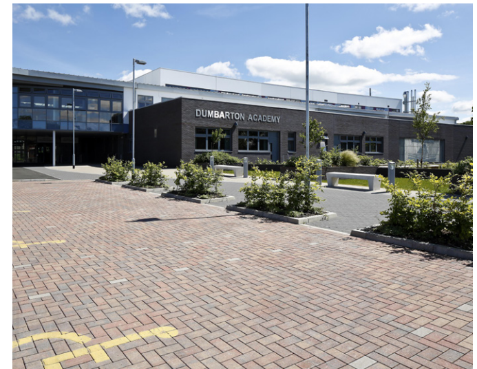
Figure 77. Permeable paving, Dumbarton Academy | Tobermore
