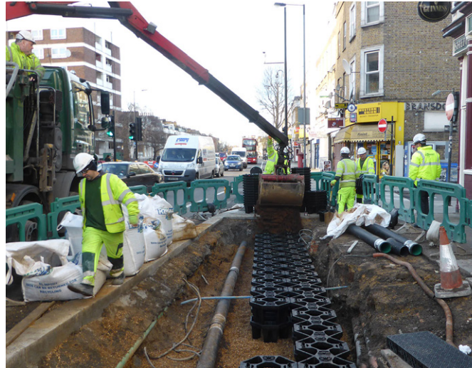
Figure 51. SuDS Tree pits under construction at Goldhawk Road | Robert Bray Associates
