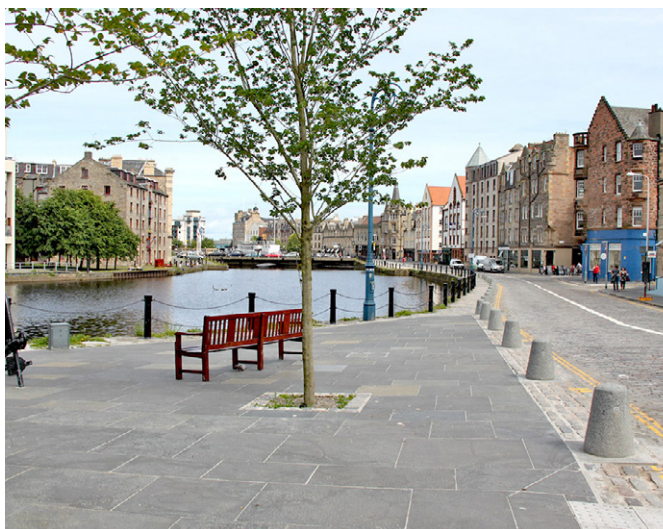
Figure 30. Leith Docks, Conservation Area | © City of Edinburgh Council
