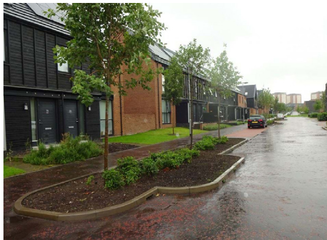
Figure 70. Street trees in rain gardens, | Sudsnet, Abertay University
