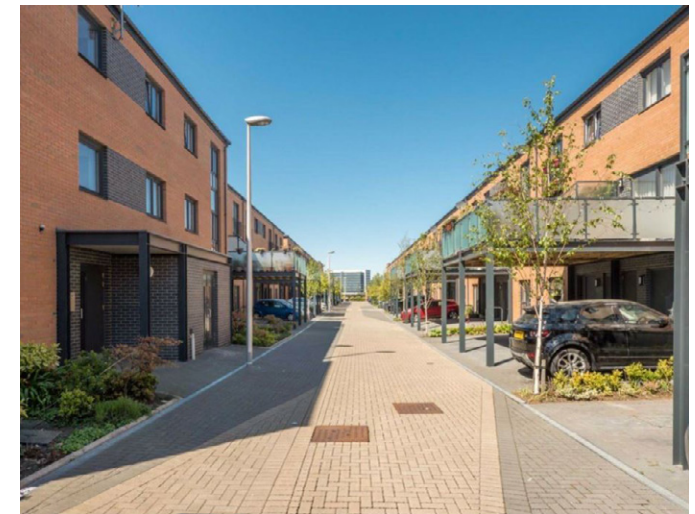
Figure 56. Permeable paving next to buildings, Stevedore Place, Leith | Atkins
