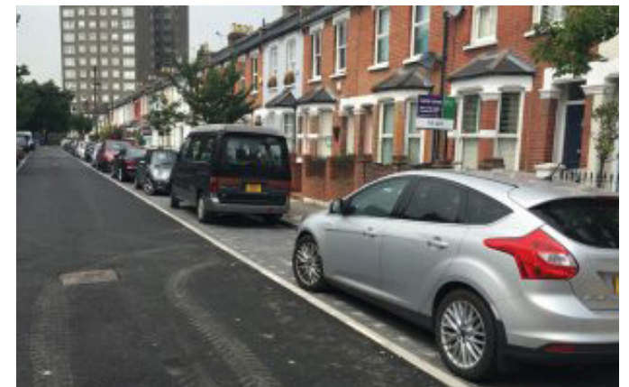
Figure 62. Completed permeable paving with geocellular storage, Mendora Road, Fulham | Atkins
