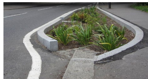
Using a filter strip to reduce pollutants
