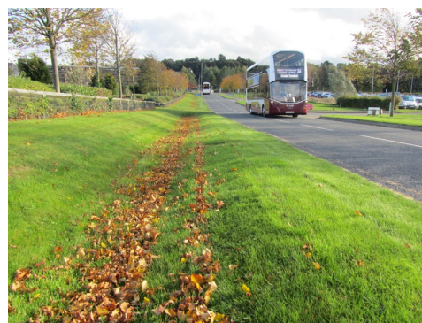
Figure 7. Swale with filter strip | RaeburnFarquhar-Bowen
