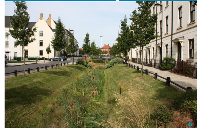
Figure 3. Upton, Northamptonshire | Susdrain, CIRIA
