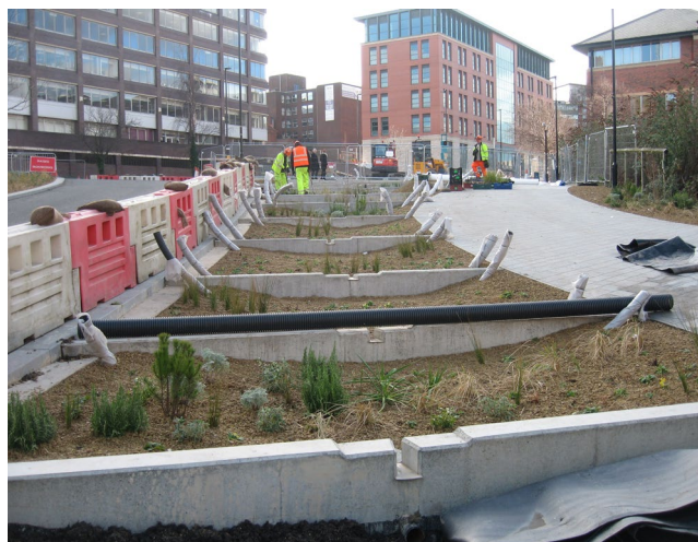
Figure 9. Swale during Construction | Sheffield City Council
