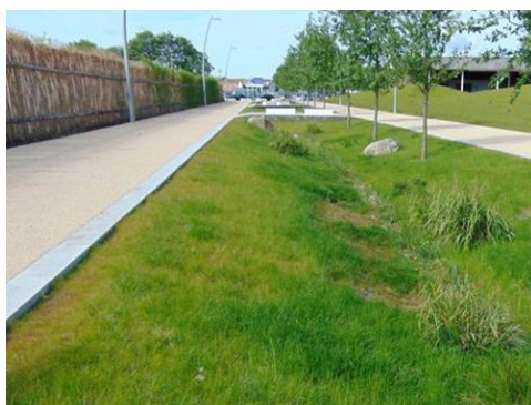
Figure 6. 'Over the edge' inlet | SNH
