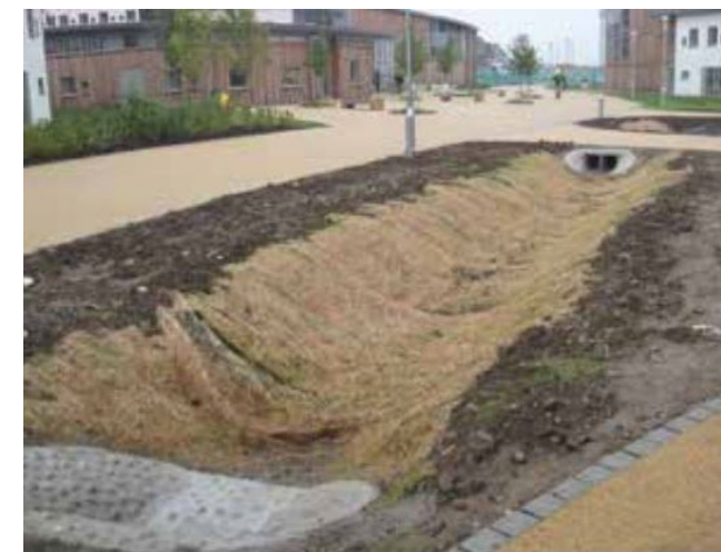
Figure 10. Swale during Construction with erosion prevention | ARUP
