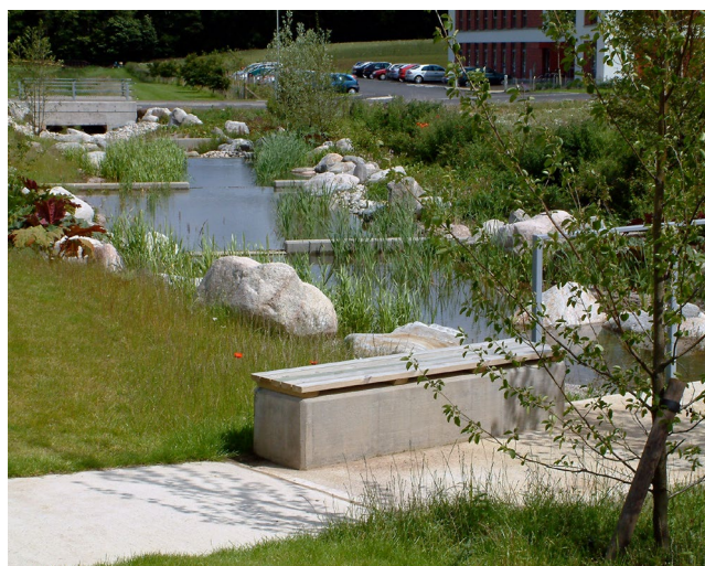
Figure 2. Wet Swale, Heriot Watt University | Raeburn Farquhar Bowen
