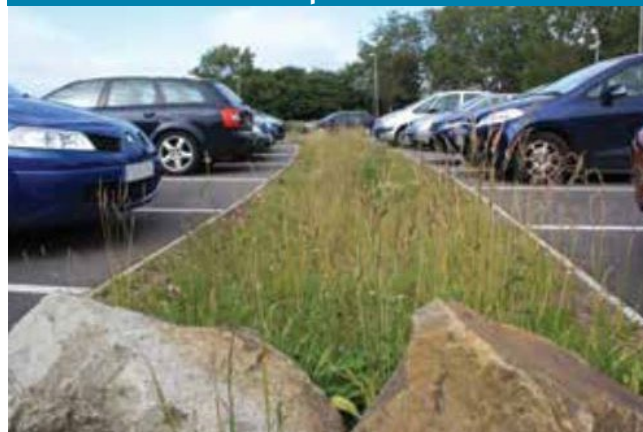
Figure 4. Swale in a car park | CIRIA
