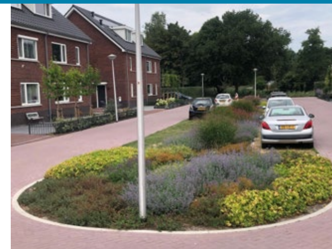
Figure 10. Rain garden under construction | Hydrorock
