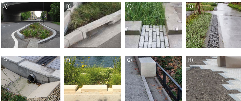
Figure 8. Examples of kerb inlets - see reference list
