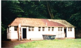
June 1999 Vandalised and neglected
