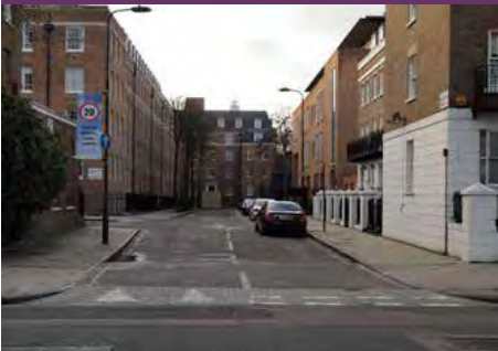
Entry Treatment with Asphalt Table
