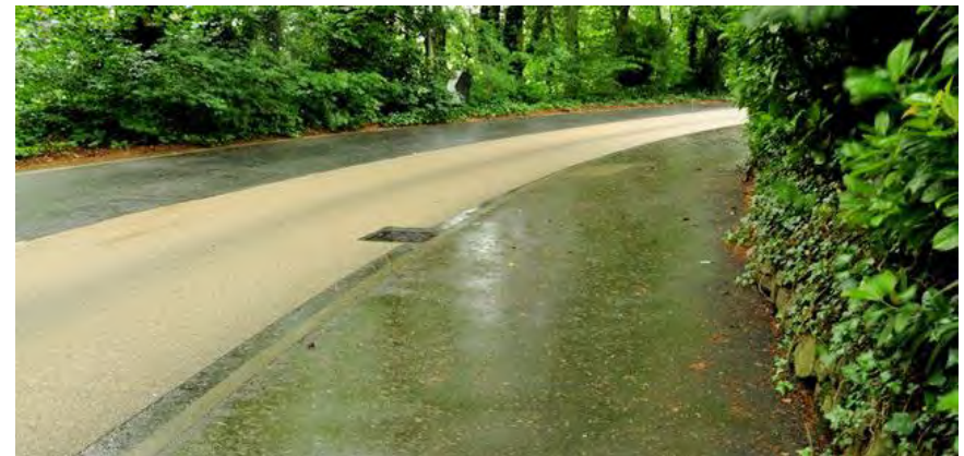
HFS on large bend in the road with wet weather conditions, Albert Bridge (2012)
