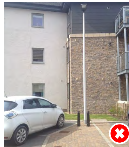
The City of Edinburgh Council: Poor positioning of street lighting, unclear whether the column is located on carriageway/footway/shared space and erecting bollards for protection from vehicles has a negative impact on street clutter.
