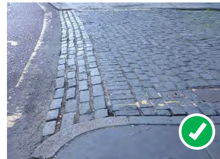
Access to historic street
