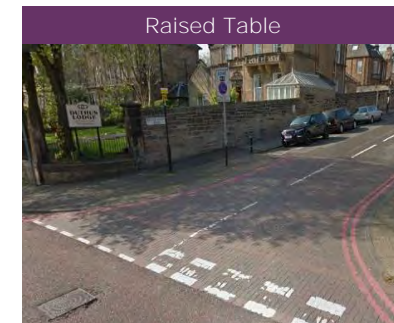
Google Maps 2017 : Raising the carriageway to create a raised table/shared surface.
