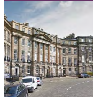
Palace frontage, Moray Place (Google Maps)
