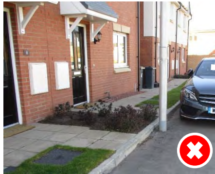
The City of Edinburgh Council: Poor positioning of street lighting, this should never be located in the carriageway space.
