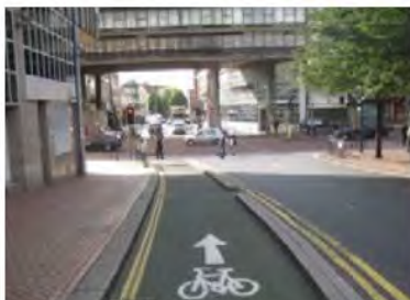
One-way contraflow cycle track on carriageway with kerb separation, Hill Street, Birmingham ( Sustrans Design Manual: Chapter 4 (2015) draft )
