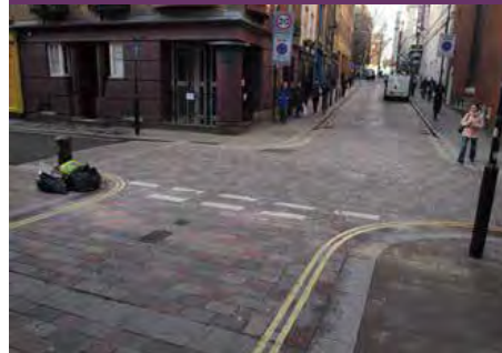
Raised Table at Junction
