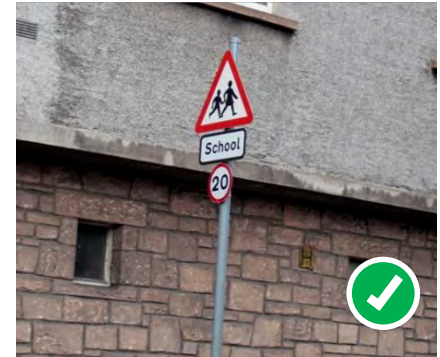
The City of Edinburgh Council: Existing pole used to accommodate new 20mph signage (small sign used) on Canongate, Edinburgh.
