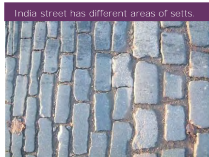
Original dolerite setts and channel with sandstone kerbing (probably Hailes).
