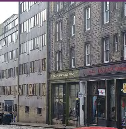
Wall mounted on St Mary's Street
