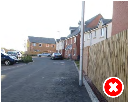
The City of Edinburgh Council: Poor positioning of street lighting, this should never be located in the carriageway space.
