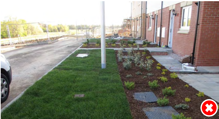
The City of Edinburgh Council: Poor positioning of street lighting, unclear to public/home owners whether the column is located in a service strip of front garden.
