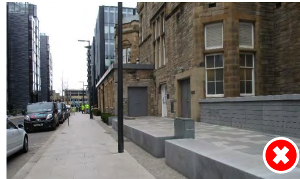
The City of Edinburgh Council: Poor positioning of street lighting, it could be placed further back in the footway so that it does not unnecessarily reduce the clear footway zone.
