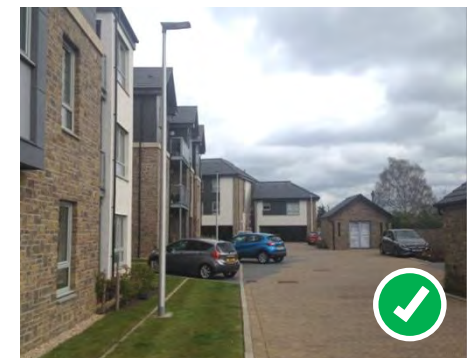
The City of Edinburgh Council: Good positioning with clear service strip area and demarcation line for ownership, also no tree/bushes planted near the columns.
