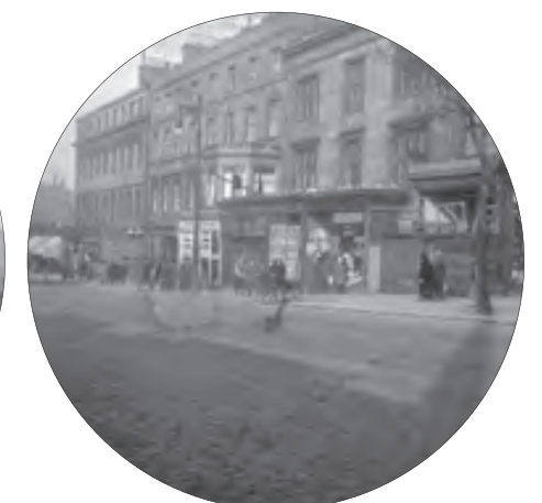
Looking north east along Lothian Road.
