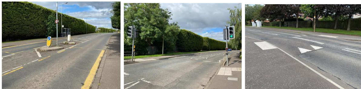
Photographs 22-24: Existing Crossings on Stirling Road
