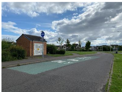
Photograph 2 and 3: Eilston Road Bus and Taxi Lane
