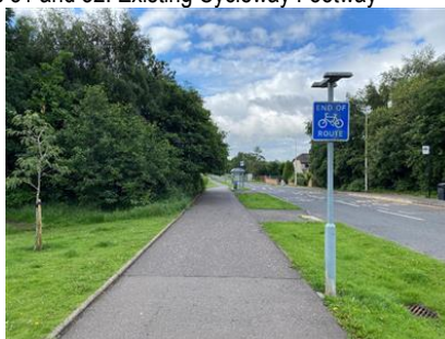
Photographs 31 and 32: Existing Cycleway Footway
