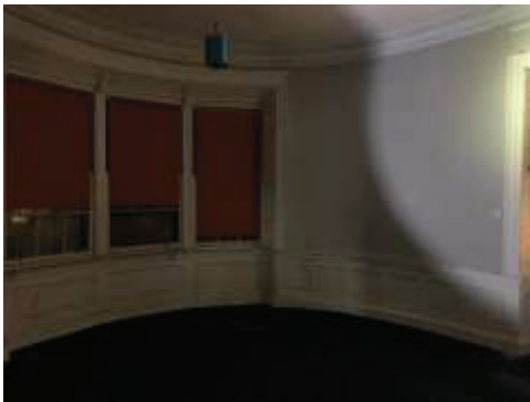
Source: DM Hall Site Inspection
