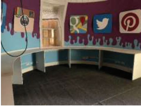
Source: DM Hall Site Inspection
