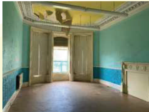
Source: DM Hall Site Inspection
