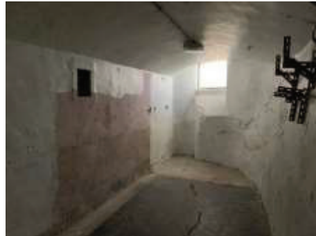
Source: DM Hall Site Inspection
