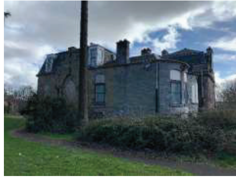
Source: DM Hall Site Inspection
