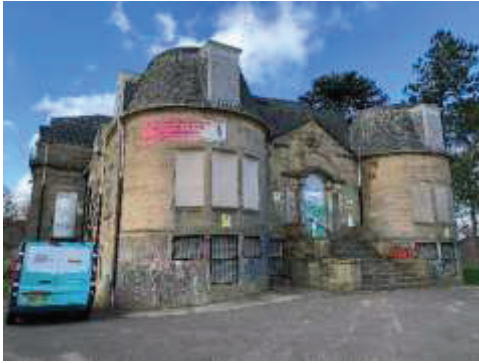
Source: DM Hall Site Inspection
