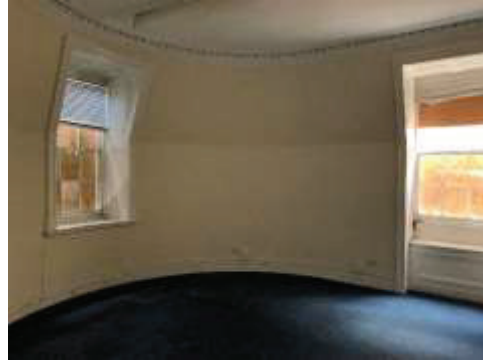
Source: DM Hall Site Inspection
