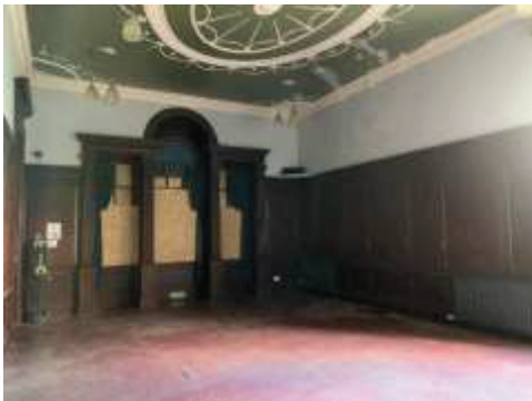
Source: DM Hall Site Inspection
