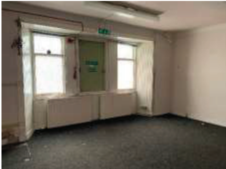
Source: DM Hall Site Inspection
