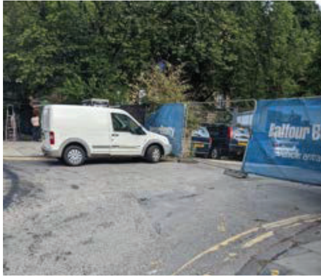
Figure 49: Ward 11- City Centre- Meadow Walk under construction
