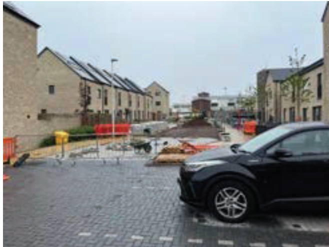
Figure 32: Ward 07- Sighthill/ Gorgie- Weir Street- Unclassified Road
