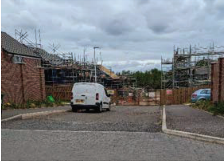
Figure 73: Ward 17 – Portobello - Nealands Road – Under construction
