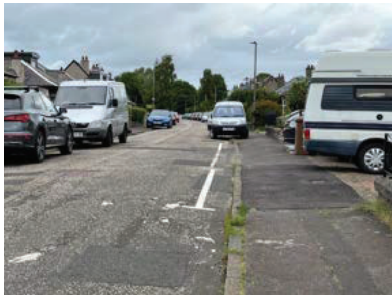
Figure 45:Ward 09- Fountainbridge- Cluster 01- Ashley Drive
