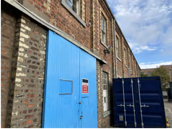
East Elevation of Lighthouse
