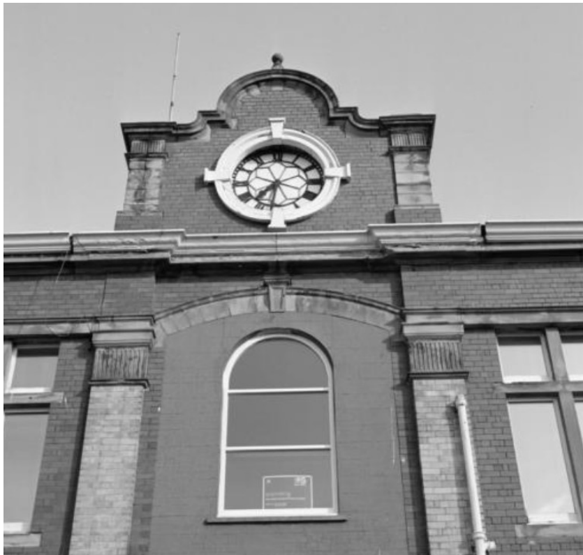
Figure 43: Clock to station building having suffered storm damage, 1998 (Canmore 2023)
