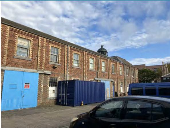
East Elevation of Lighthouse
