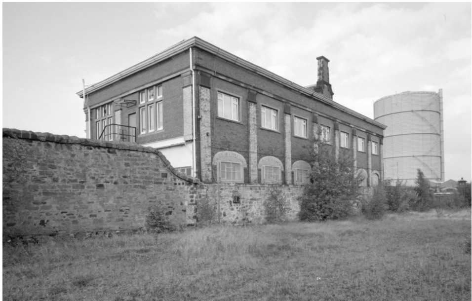
Figure 42: Rear of Station Building, 1998 (Canmore 2023)
