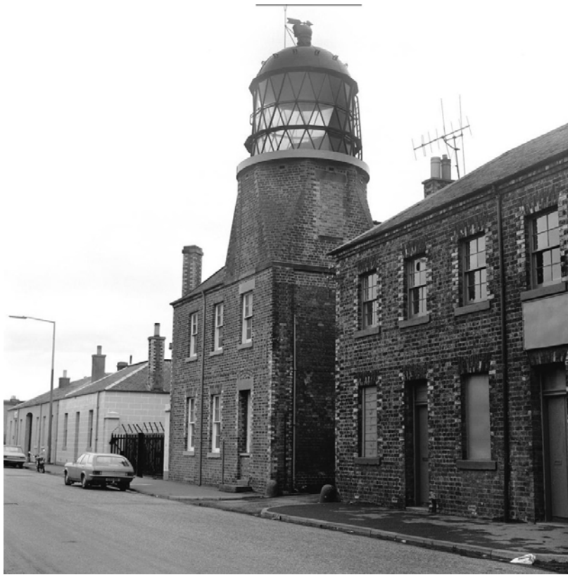
Figure 37: West Harbour Road, Granton 1979 (Canmore 2023)
