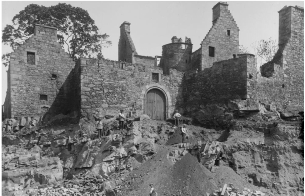
Figure 25: View of men digging beneath Granton Castle in 1890 (Canmore 2023)
