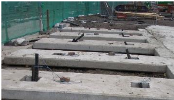
Figure 24: Raft system installation and completed project, Glasgow
