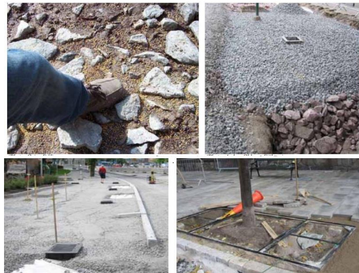
Figure 25: Urban tree pit installation sequence in Stockholm
