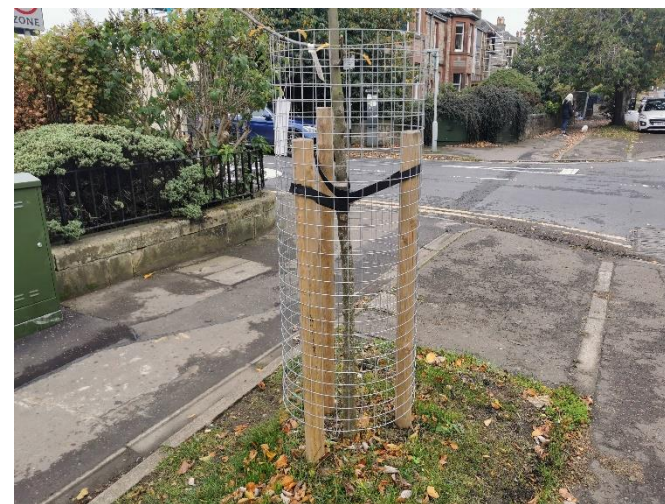
Figure 32: Triple stake and weldmesh guard system
