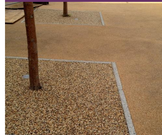
Figure 28: Resin surface treatment
