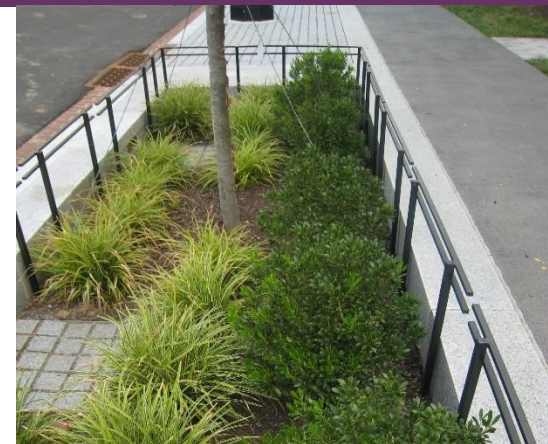
Figure 22: Tree with open pit/trench and underplanting.
