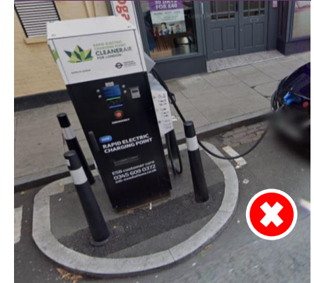
Figure F8.9 - Chargepoints on raised kerbs with poorly placed bollards make wheelchair access difficult
