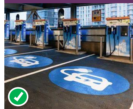
Figure F8.18 - Bulky rapid chargers are better suited to off-street locations
