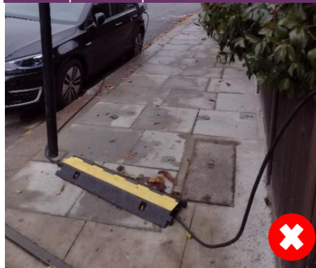
Figure F8.24 - Even with matting over the cable there is an unacceptable trip hazard
