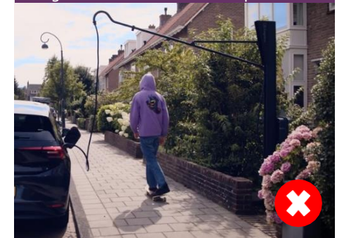
Figure F8.25 - Charge arm: home charger elevated to avoid trip hazards
