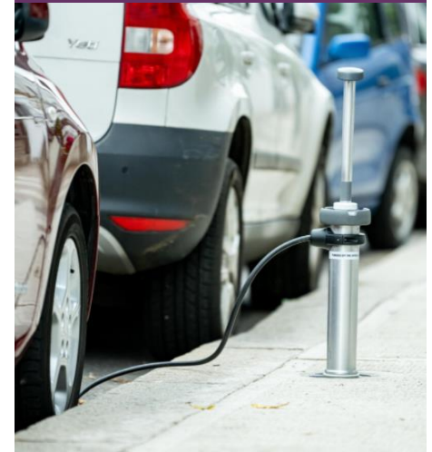
Figure F8.11 - Retractable or slimline chargepoints in colours that match existing street furniture
