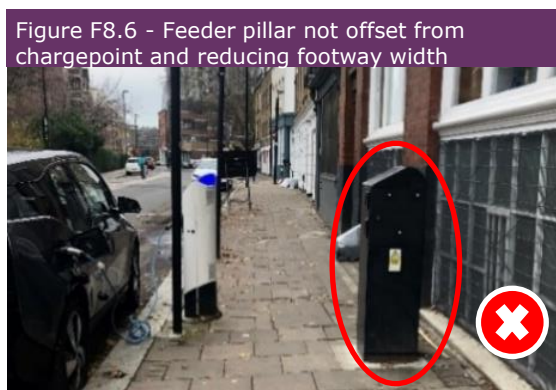
Figure F8.6 - Feeder pillar not offset from chargepoint and reducing footway width Google Streetview
