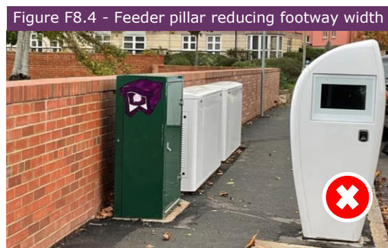
Figure F8.4 - Feeder pillar reducing footway width Google Streetview
