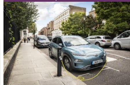
Figure F8.21 - Satellite bollard positioned between two bays
