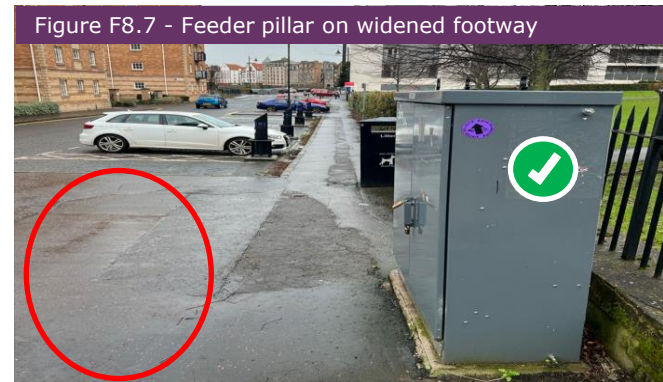
Figure F8.7 - Feeder pillar on widened footway City of Edinburgh Council
