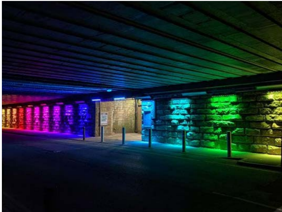
Photo : Mirfield Station Underpass www.studiotech.co.uk
