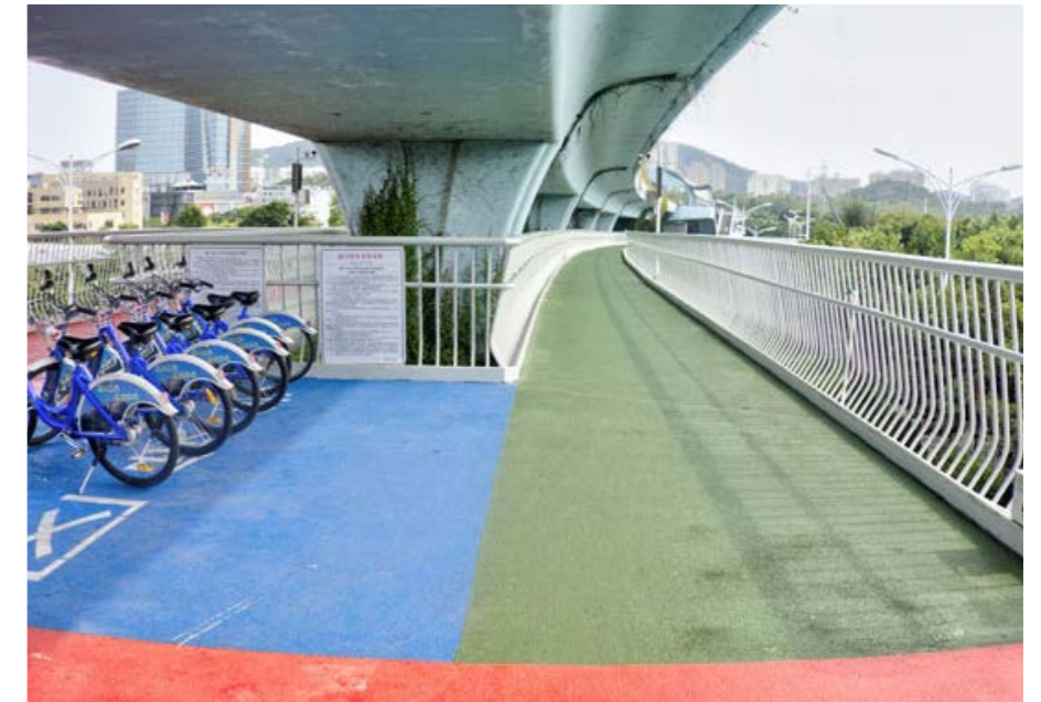
Photo : Using surface colour to articulate active travel provision - Bike Skyway, Xiamen https://thecityfix.com/blog/china-elevates-bike-lanes-to-a-new-level-mark-
