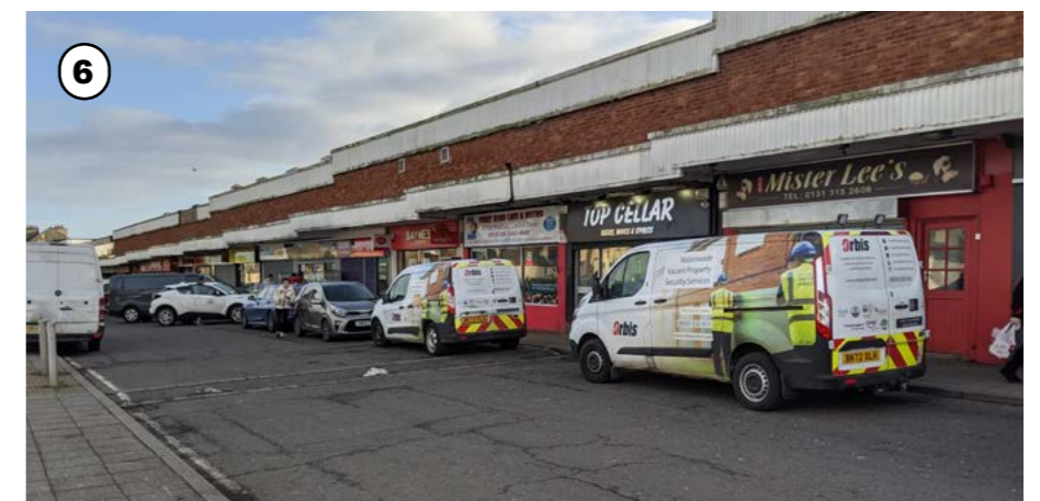
Raised crossing point is not clear or distinguishable from the carriageway space, resulting in illegal parking. There can be a high turnaround of parked vehicles, particularly during lunchtime (the time this photo was taken) as the shopping centre includes a number of cafe and takeaway units.
