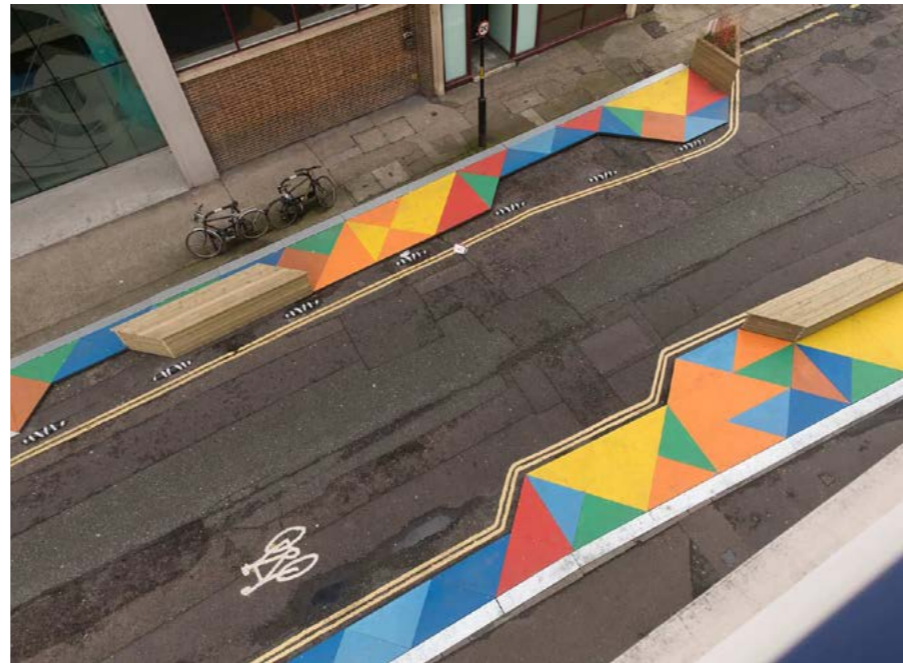
Photo : Creating buildouts using colourful modular units - Bankside Boardwalk, Bankside, London https://betterbankside.co.uk/bankside/urban-forest/bankside-boardwalk/
