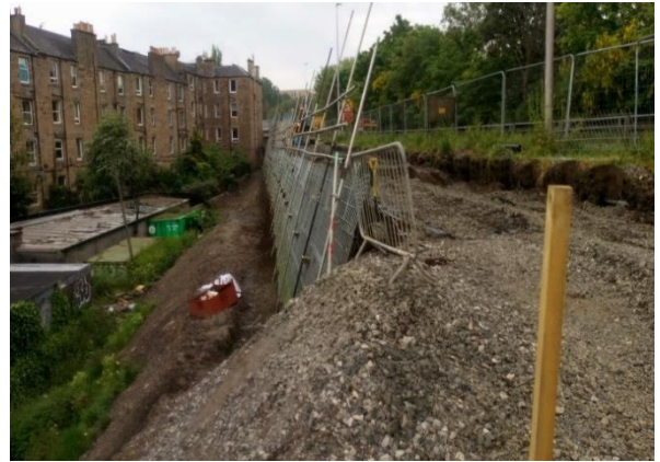
Reinforced slope beside Dalry Road Bridge
