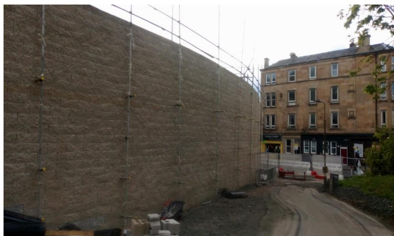
Reinforced earth block wall Dalry Park
