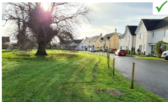
Figure 5. Roadside swale | Abertay Univeristy
