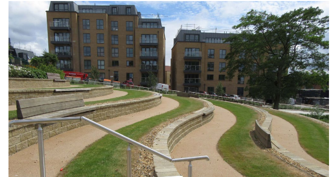
Figure 13. Park, Millbrook Park | ARC New development at Mill Hill in Borough of Barnet, London has utilised the steep topography across the site to integrate the SuDS treatment train with new green spaces as part of creative placemaking.
