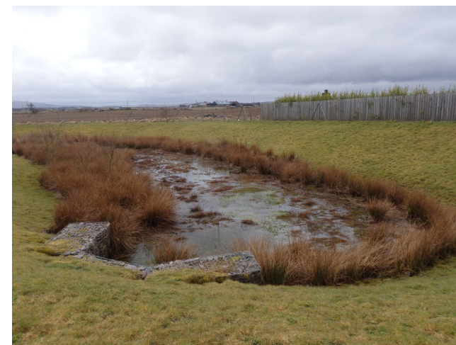
Figure 31. Gabion Inlet, Pitblae | Abertay Univeristy
