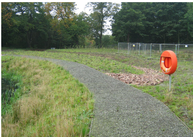
Figure 40. Lowered bank at footpath and overflow channel | Abertay University
