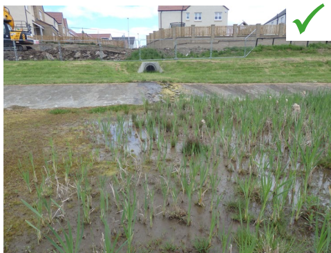
Figure 21. Sediment Forebay, Bellsdyke | Abertay Univeristy
