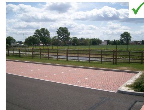
Figure 24. Permeable paving | Abertay Univeristy
