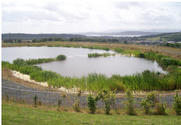
Figure 15. Forebay, Dunfermline | Abertay Univeristy Newly constructed pond with forebay, Dunfermline.
