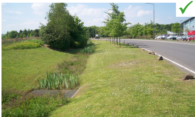
Figure 4. Swale | Abertay Univeristy
