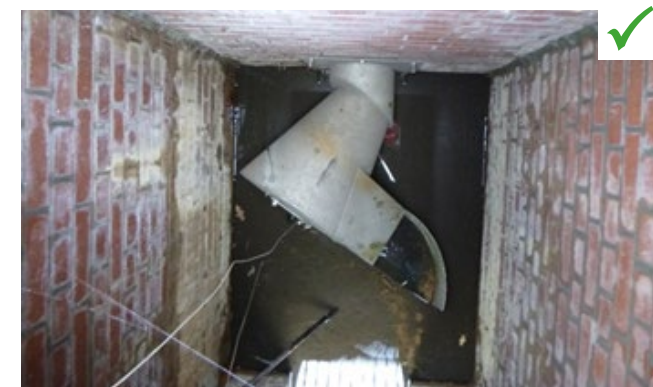
Figure 35. Vortex Flow Control | Abertay University
