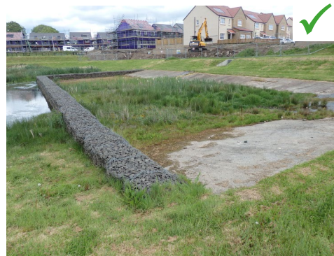
Figure 22. Sediment Forebay, Bellsdyke | Abertay Univeristy
