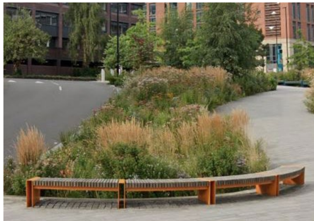
Figure 12. Swale constructed on a slope | Sheffield City Council
