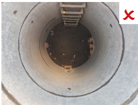
Figure 17. Sump full at manifold | Abertay Univeristy
