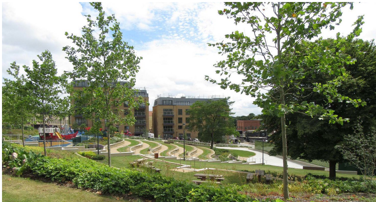
Figure 9. Swale constructed on a slope, Millbrook Park | Arc
