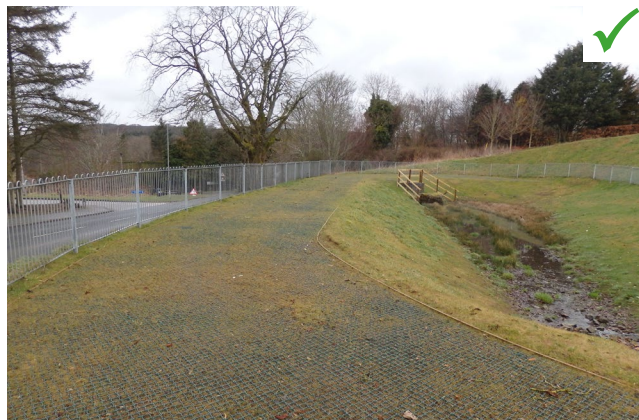
Figure 27. Grasscrete access track | Abertay University
