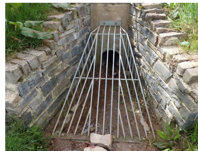
Figure 32. Stone facing headwall | Abertay University
