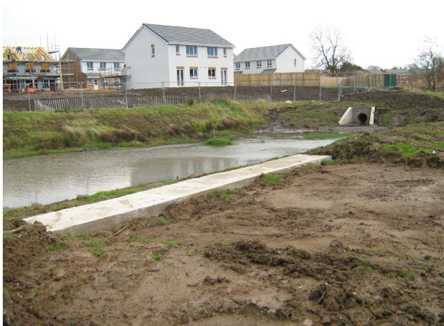
Figure 41. Concrete spillway weir under construction in west of Scotland | Abertay University
