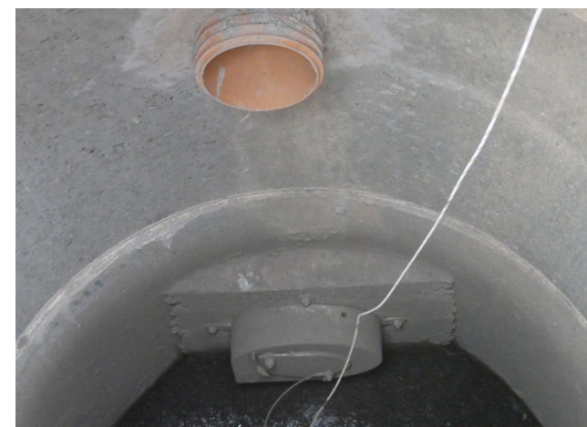
Figure 43. Internal overflow above VFC | Abertay University
