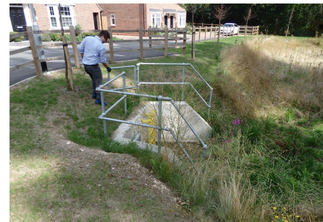
Figure 8. SuDS site inspection | Abertay University
