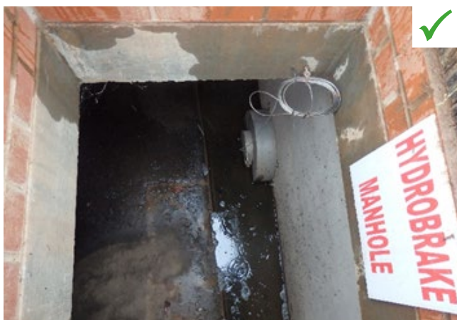
Figure 33. Vortex Flow Control | Abertay University
