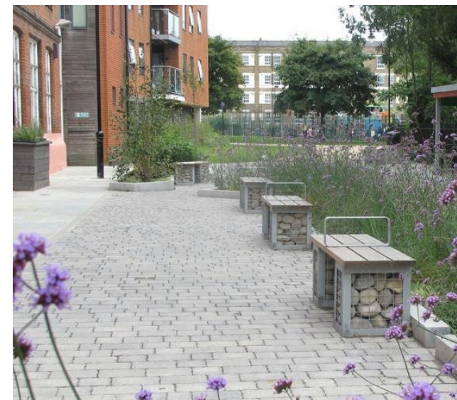
Figure 20. Permeable Paving, Derbyshire Street Tower Hamlets | Mayor of London Assembly
