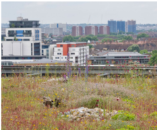
Figure 8. Biodiverse green roof on PWC 7 More London | Dusty Gedge
