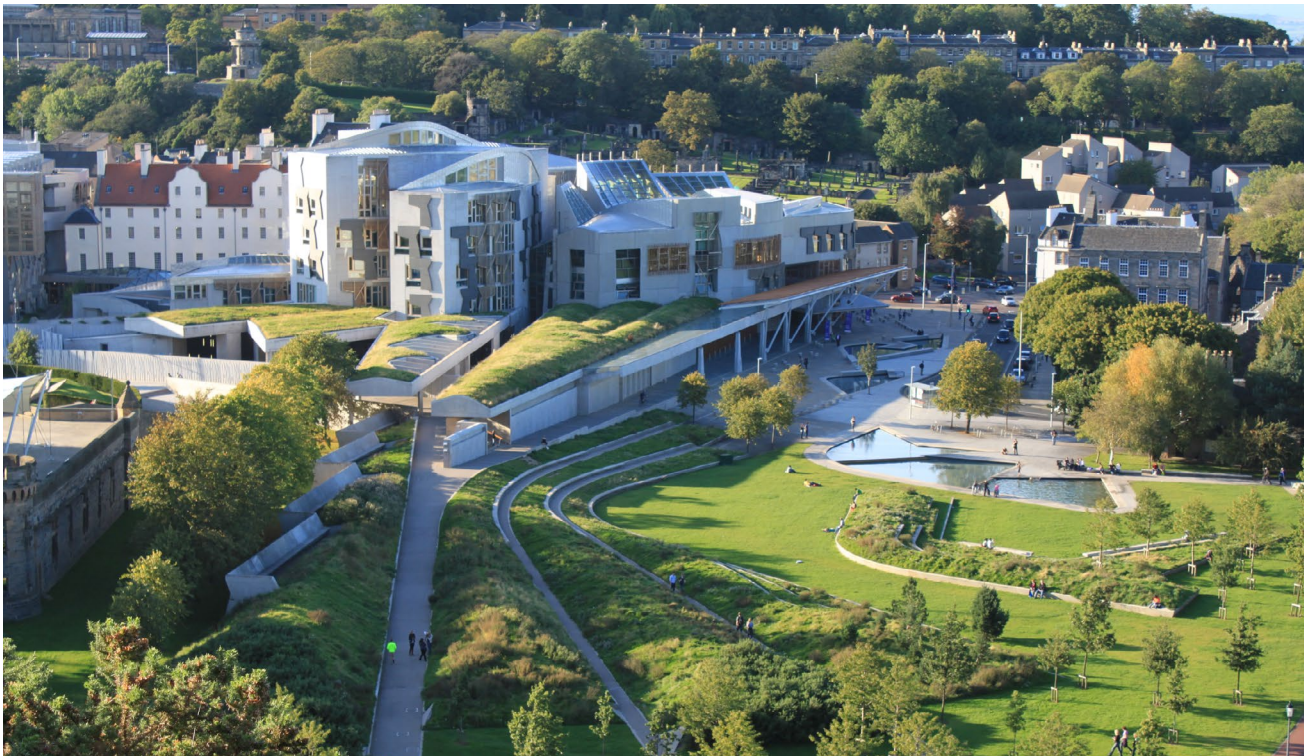
Figure 1. Edinburgh Parliament Building with Extensive Green Roof | Mark Longair
