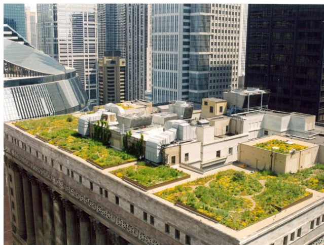
Figure 15. Chicago City Hall retrofit living roof | Farr Associates
