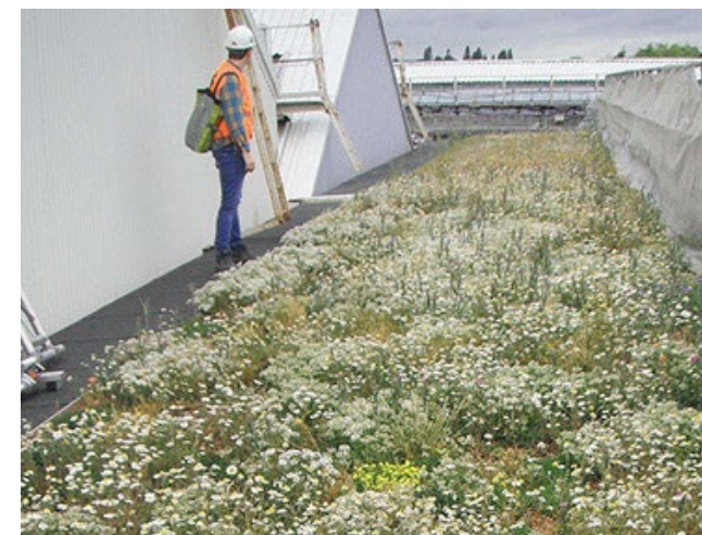
Figure 28. Ruislip Tube Depot | Susdrain
