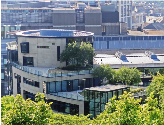
Figure 29. Intensive roof, Greenside Row, Edinburgh | Atkins
