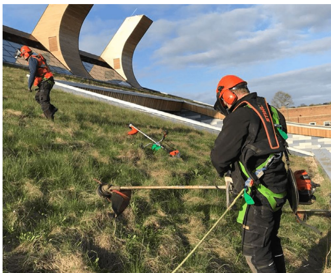
Figure 17. Maintaining a Living Roof | ICB Projects
