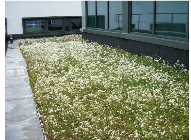
Figure 33. Extensive Green Roof | Edinburgh Vet School (©. Bauder)
