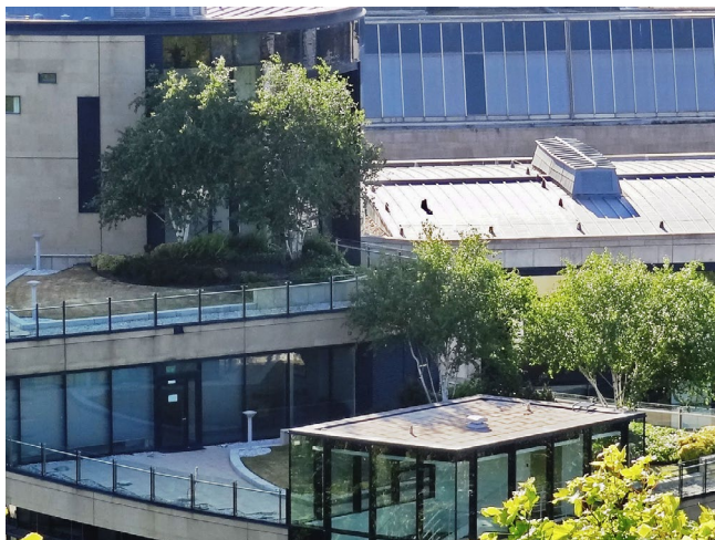
Figure 5. Intensive roof, Greenside Row, Edinburgh | Atkins
