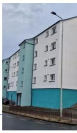
**Before** - blocks of flats in Wester Hailes showing the roof in poor condition, render spalling and cracking to the building fabric.
