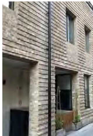
Brick with texture in detailing
