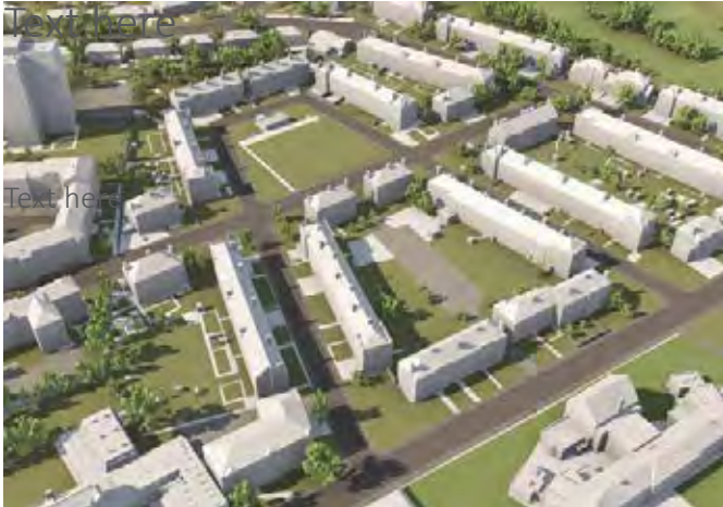
Restalrig - 1940s 3 storey flatted buildings
