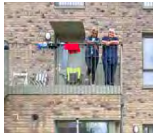
Leith Fort - Port of Leith Housing Association (Collective Architecture and Fraser/ Livingstone Architects
