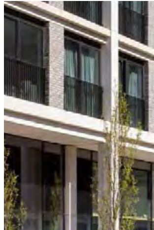
Concrete and brick
