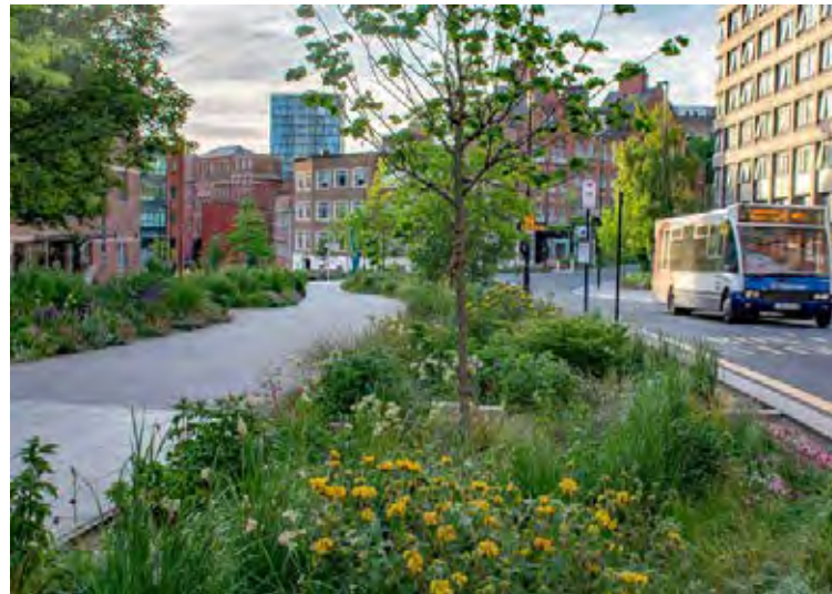
Sustainable drainage and street greening- Sheffield
