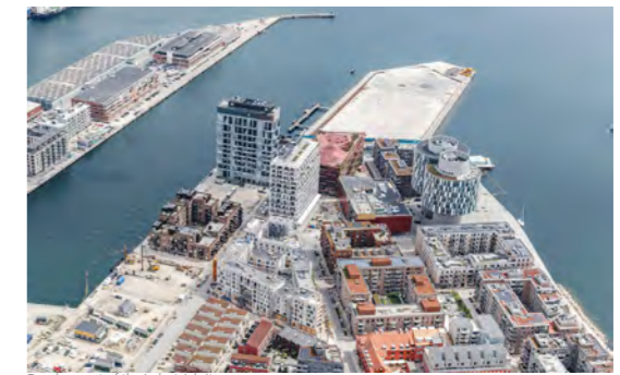
Development of the industrial site
