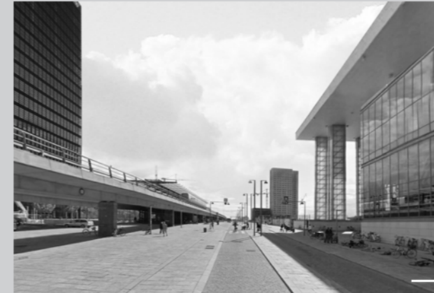
Existing - empty space beneath metro
