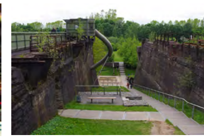
Landscaping work to link industrial remains
