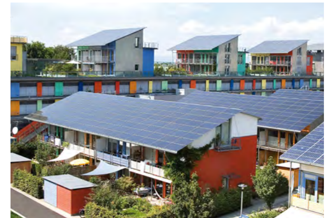
Extensive solar panels on living units
