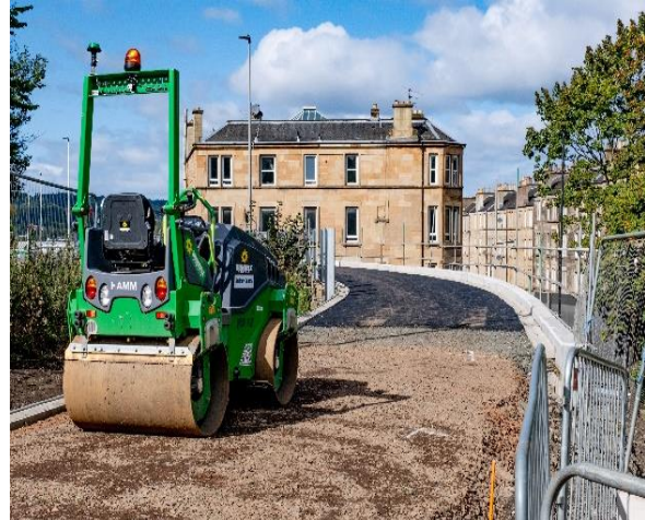
Path surfacing underway over Dalry Road Bridge
