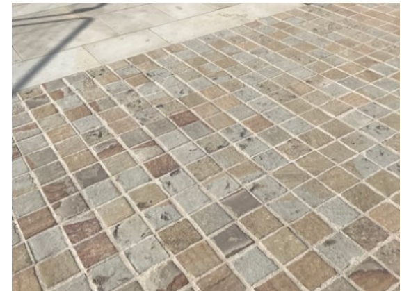
Above: a building trim detail, formed by smaller paving units, could be utilised as a threshold indicator.
