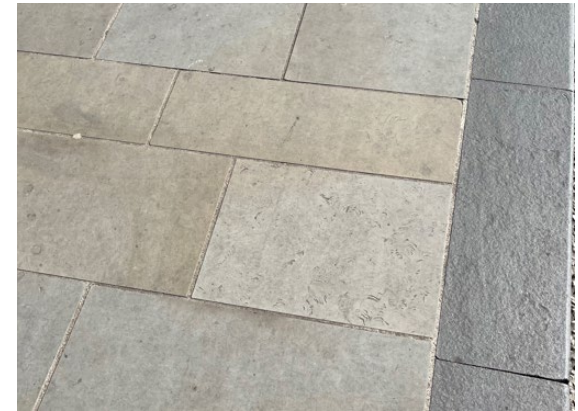
Above: use of wide Whinstone or dark granite kerbs with Sandstone flagstones
