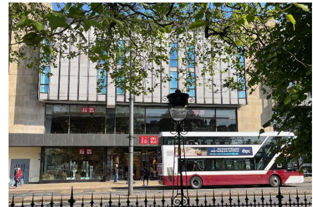
Image above: the completed redevelopment at 64 Princes Street, a category B Listed building and home to Edinburgh's Uniqlo store.
