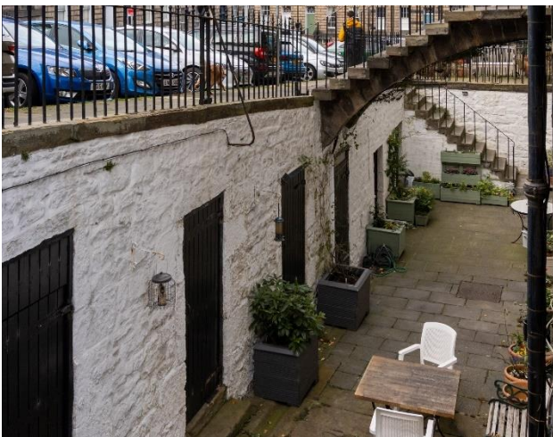
Basement area with cellar storage
