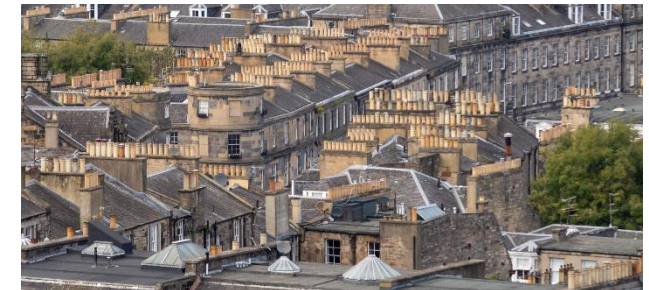
Chimney details on Edinburgh roofscapes
