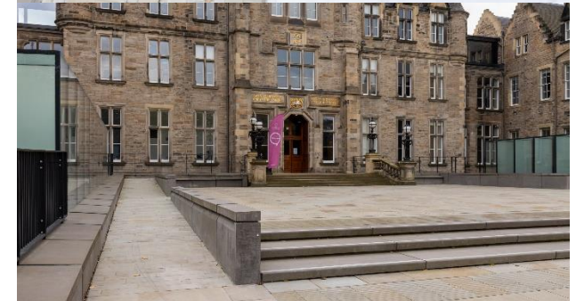
Ramp at Edinburgh Futures Institute. Original stone staircase moved forward to accommodate ramp. Category A listed, LB30306, 31/05/1994
