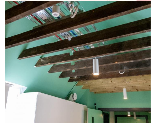
Surface mounted services behind original roof beams
