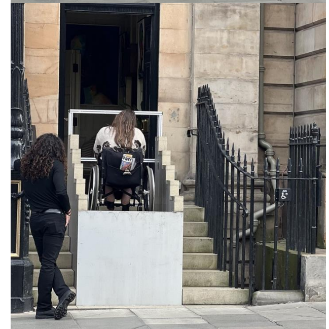
Hidden platform lift in use. Stairs fold back to form the platform and the lift provides level access for the user.
