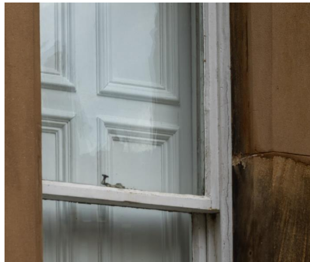
Timber window shutters
