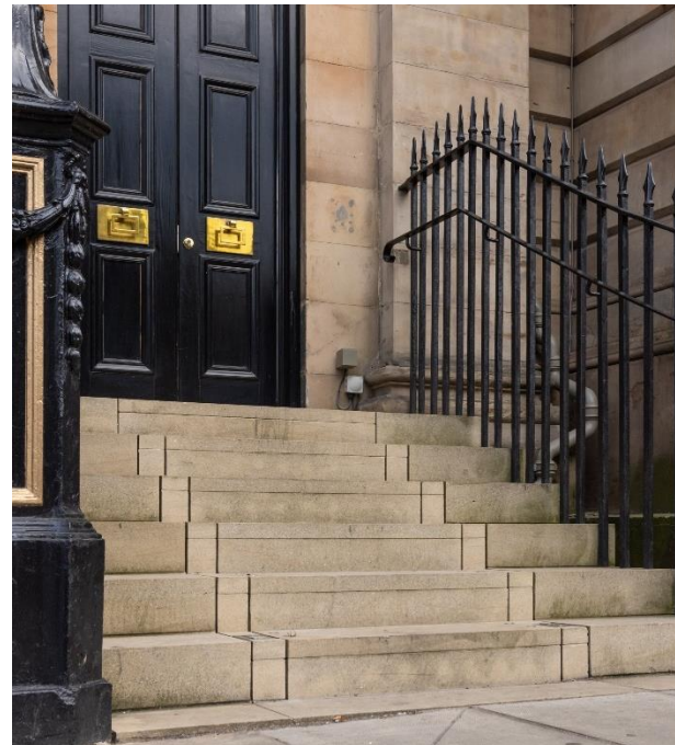
Hidden platform lift at Gleneagles Townhouse Hotel, Category A listed, LB29707, 13/04/1965
