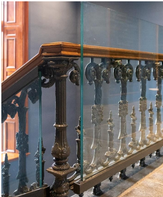
Figure 1 Safety barriers retrofitted to original features
