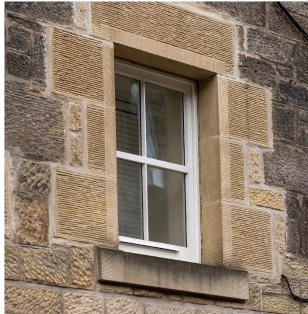
Matching stonework around new window
