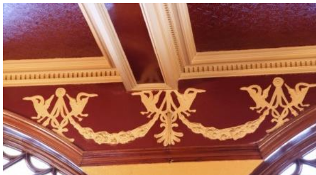
Decorative ceilings ©Historic Environment Scotland
