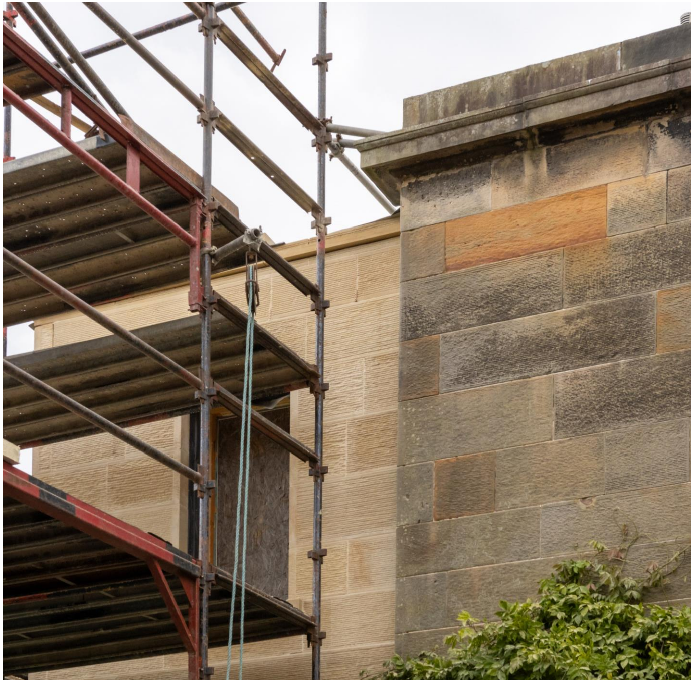
Side extension with matching stonework on a traditional building
