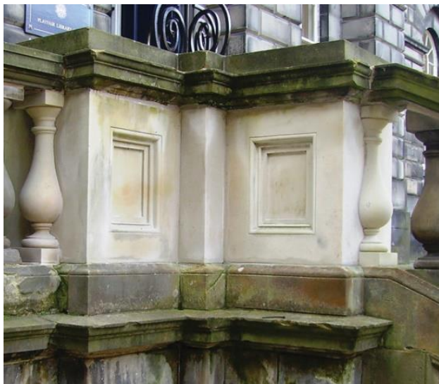
Example of stone repair matching details
