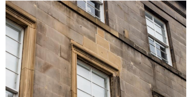
Indent stone repair and matching window details
