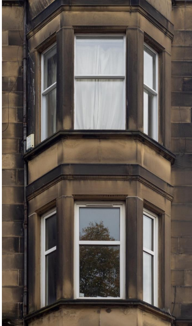
Visible differences between timber sash and case windows and uPVC windows
