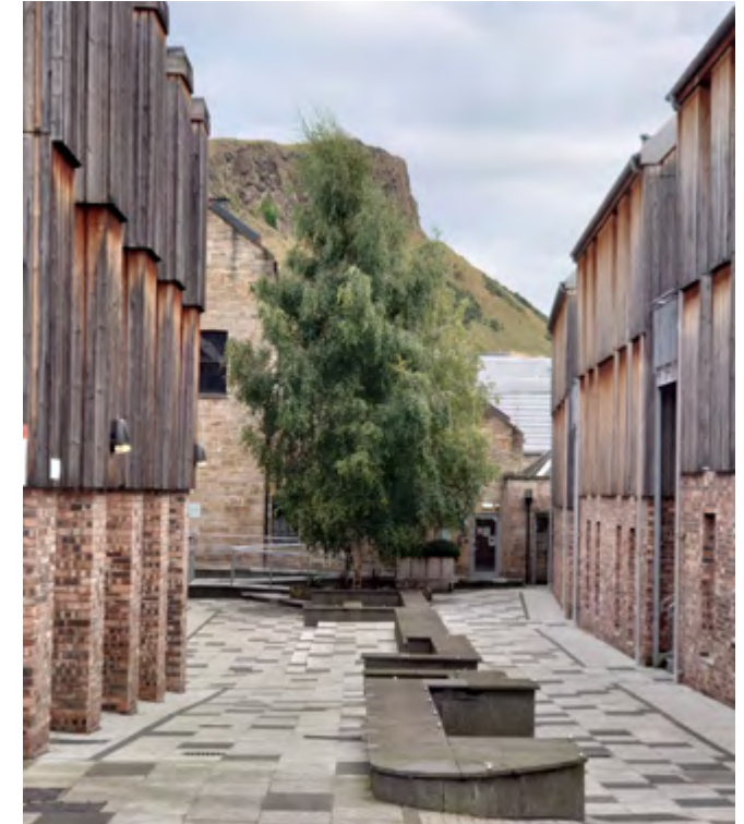
Timber informed by historic context: Sugar House Close - Timber cladding to the upper floors of this development off the Royal Mile takes a cue from the pattern of external finishes on adjacent historic buildings.
