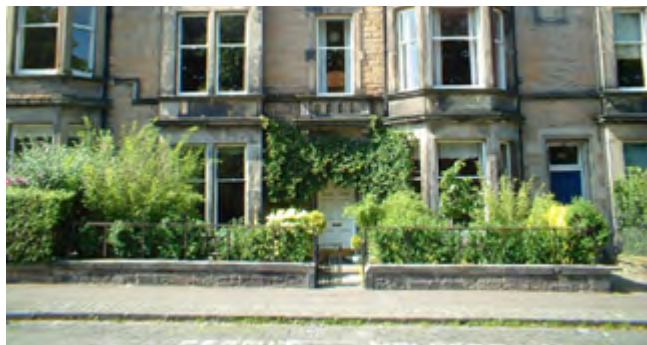
Active frontages and housing—Marchmont Tenement - Traditional tenements (above) have main doors directly into ground floor flats which maximises activity on the street and help ensure front gardens are used.
