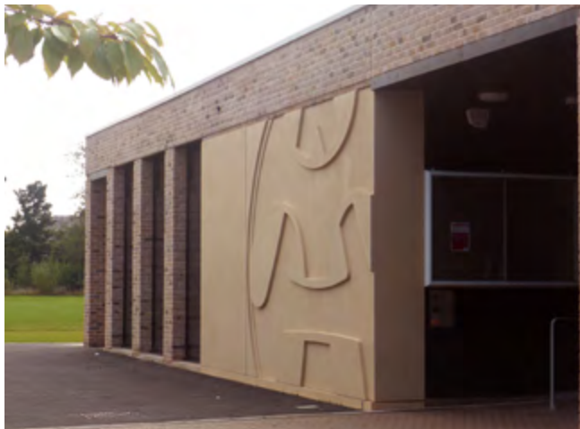
Concrete used sculpturally to contrast with brick - At Bangholm Outdoor Centre, precast concrete with the school badge creates an attractive contrast to the texture and colour of the brickwork, while marking the entrance of the centre.
