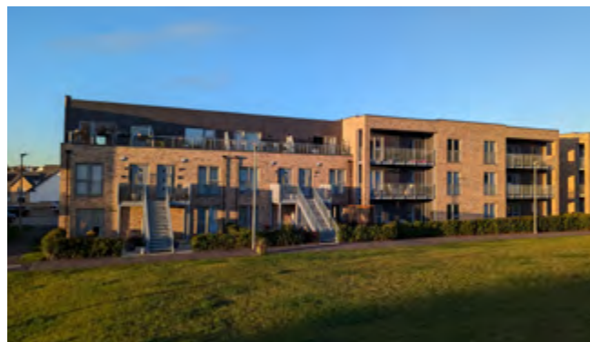
Density with a mix of housing types - Cammo includes a mix of flats, colony houses, townhouses, terraced and detached houses.
