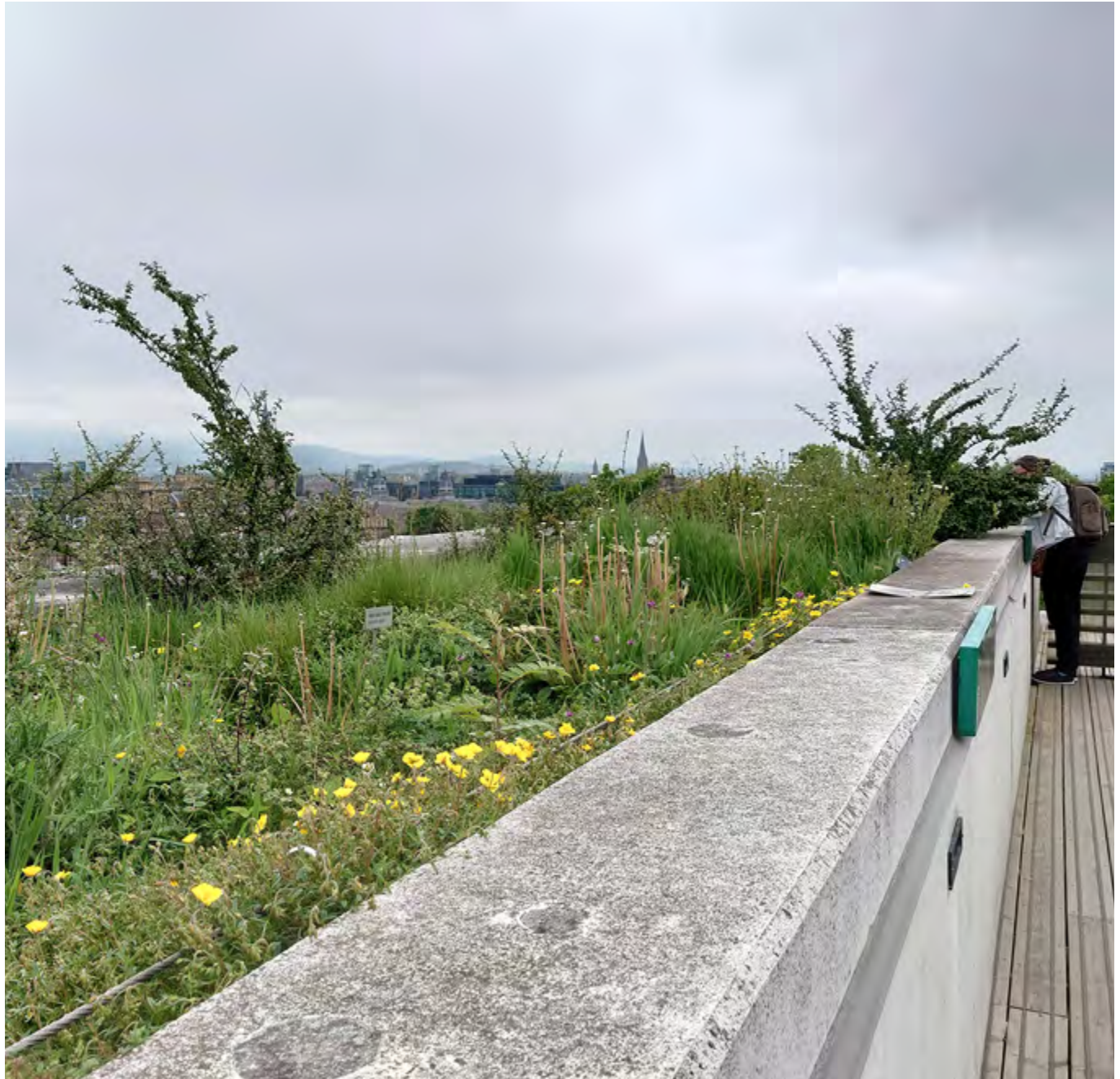
Rooftop planting to reduce risk - The intensive planting on the rooftop of the National Museum of Scotland provides an attractive edge, while also delaying or deterring anyone from accessing the roof edge.
