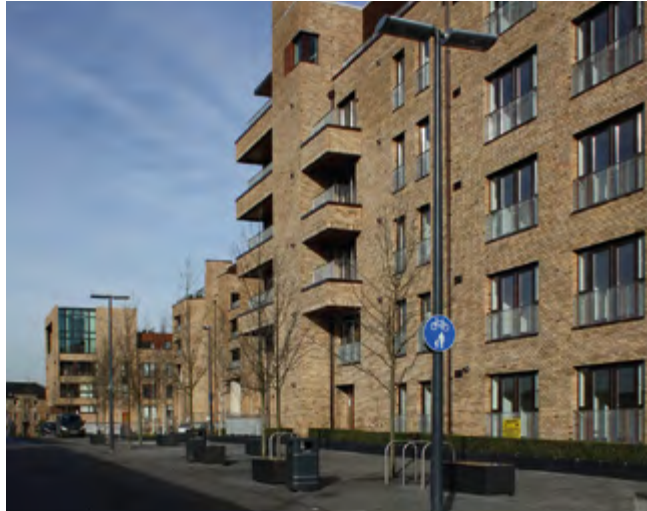
Modern use of brick in an historic environment: McEwan Square, Fountainbridge - Brick has been used to integrate this development into its historic surroundings. The development is overtly contemporary in its appearance. The colour of bricks was chosen to harmonise with the stone of the adjacent tenements. Combined with the vertical emphasis to the window and the building's scale, the material choice has helped ensure this development adds to Edinburgh's sense of place.
