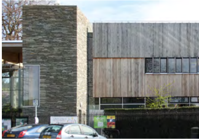
Careful detailing: Arboretum Place - The timber cladding overhangs cladding on lower levels of the building. This helps shed water from its surface, and protects it from adverse weathering.
