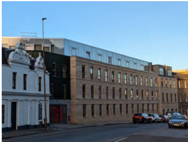
Recessed top floor, Montrose Terrace - The top floor of this student accommodation scheme has been set back. This means that the dominant height of the front façade matches the eaves height of the adjacent tenements.
