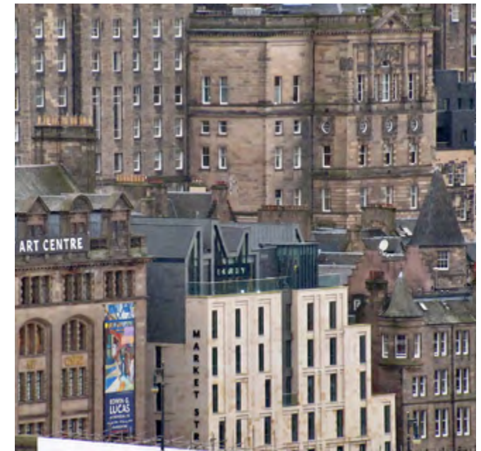
Roofscape that responds to context - The roof of this hotel on Market Street has been designed to reflect the form of the roofscape behind it.
