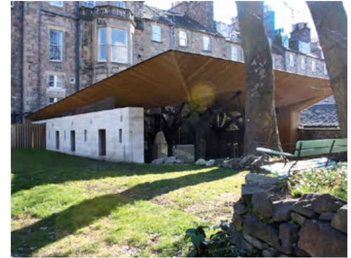
Frameless glazing: Chapel of Saint Albert the Great, George Square Lane - Glazing is used to create the effect of a floating roof on this distinctive Catholic Church.
