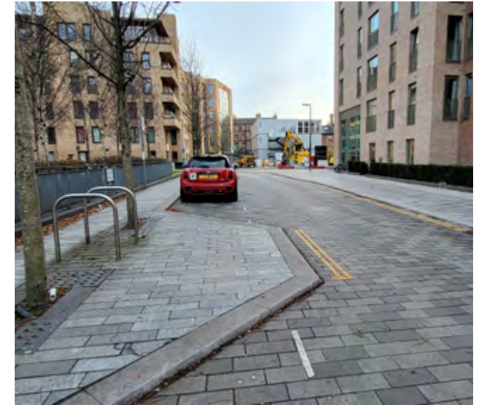
Streets incorporating parallel on-street parking - Prince Regent Street provides parallel parking on-street, interspersed with build-outs. It is acceptable to assume informal 'give and go' between parked cars, providing relatively narrow residential streets.
