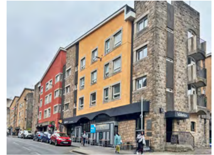
Sensitive refurbishment can enhance efficiency and heritage - These flats on Canongate were refurbished by Edinburgh World Heritage in partnership with City of Edinburgh Council. The B-listed flats were designed by Sir Basil Spence. They were refurbished to improve the operational efficiency, while respecting and enhancing the cultural significance. An MVHR system was installed, along with improved insulation and building repairs. The windows were replaced with double glazed windows that also reinstated Spence's original design
