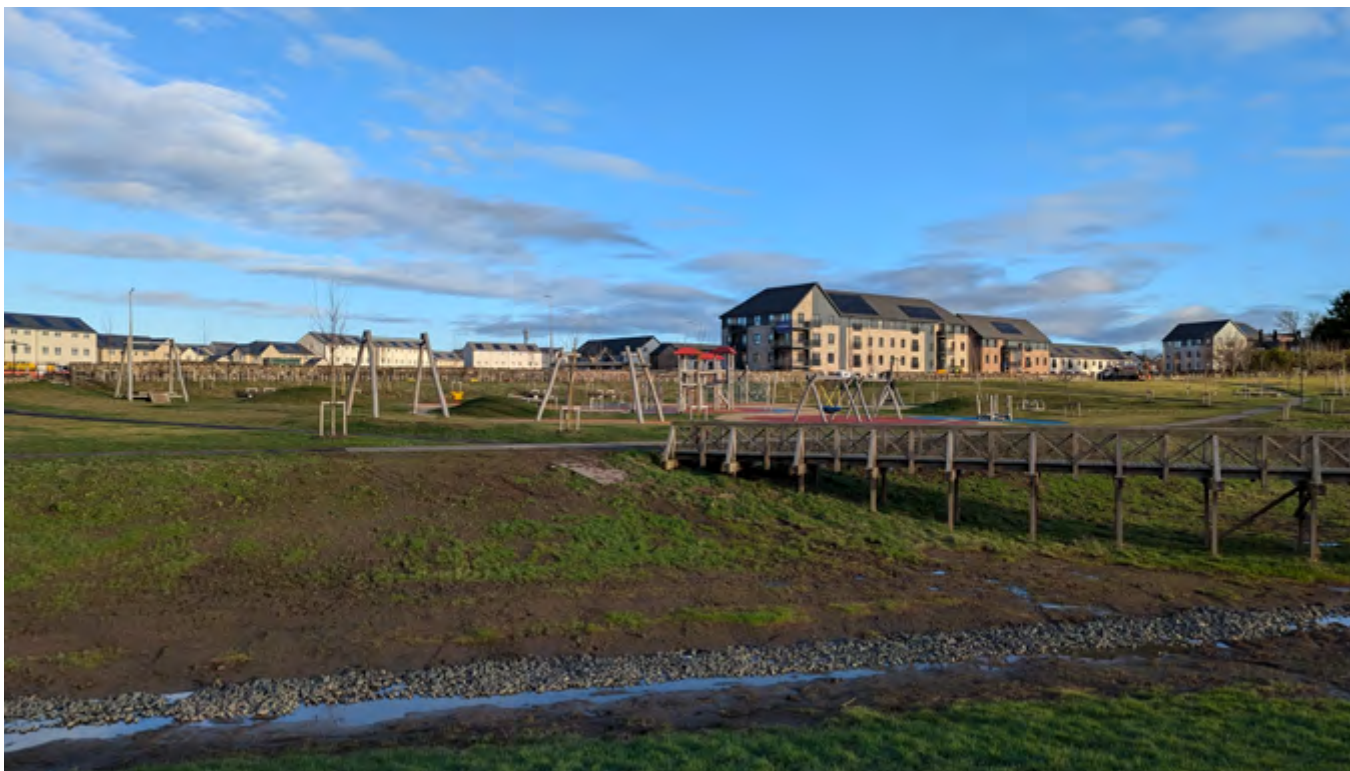
SuDS integrated from the outset - Sustainable rainwater management was considered from early in the design process of Meadowfield Park in West Craigs. It forms an integral part of the wider park. The park has been designed with a raised timber walkway and wildflower meadow planting.
