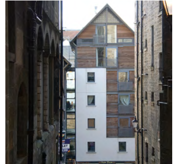
Positive contrast: Old Fishmarket Close, off High St - The use of render and timber contrast positively with surrounding stone buildings.
