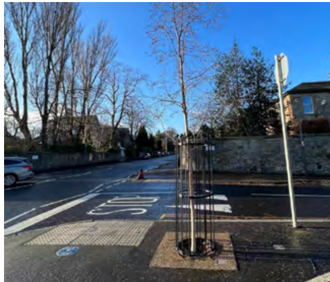
Raised junctions with narrow corner radii - Tighter corner radii at side streets can create shorter crossing distances, space for placemaking and SuDS e.g. street trees. Raising the carriageway to footway level slows traffic, making it easier and safer for pedestrians to cross.
