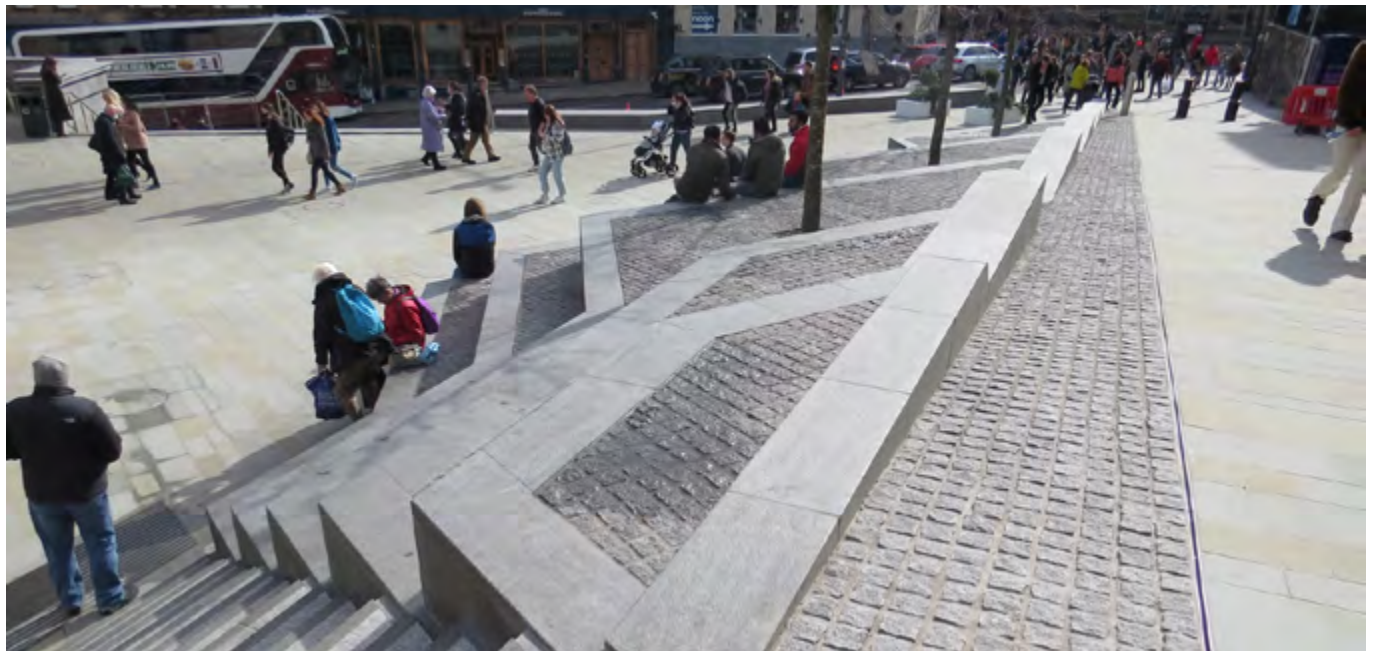
Providing high quality hard landscape: St James Quarter - This new public space off James Craig Walk connects the St James Quarter entrance to the east end of Princes Street. It features sandstone paving, granite seating terraces, and street trees.
