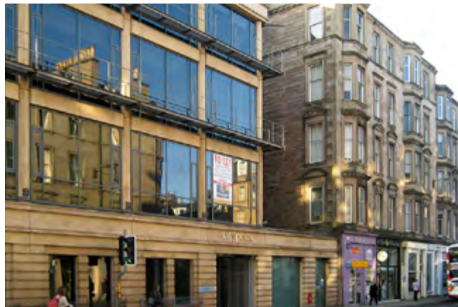
Including a set back from a gable: Haymarket Terrace - The upper floors of the modern office are set back from windows on the tenements' gable. This allows some daylight to reach the windows, but importantly maintains the street frontage.
