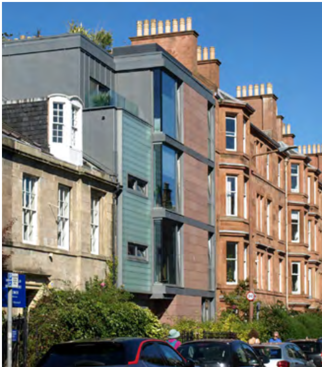
Matching heights in tenement streets - It is important that new buildings on tenement streets have similar heights to their neighbours. This modern building is designed so that the height of its main walls matches the eaves heights of the adjacent tenement.
