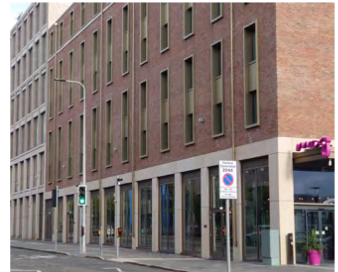
Modern use of brick in a historic setting - This Fountainbridge hotel was built using a modular off-site construction system and clad in brick to present a contemporary aesthetic that references the area's industrial heritage.
