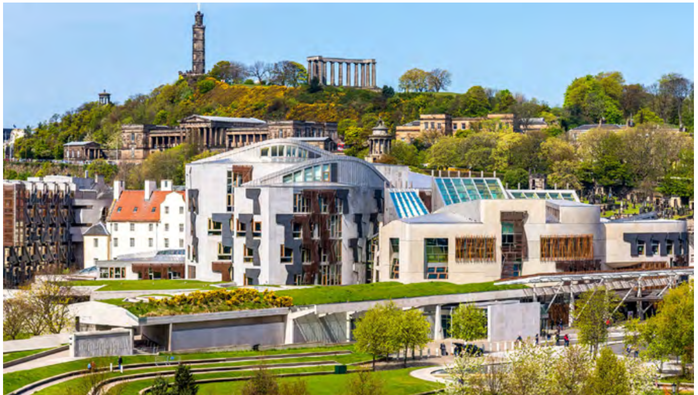
Providing a high quality external environment: Scottish Parliament - The landscape design creates an inspiring space that responds to the context © Getty Images
