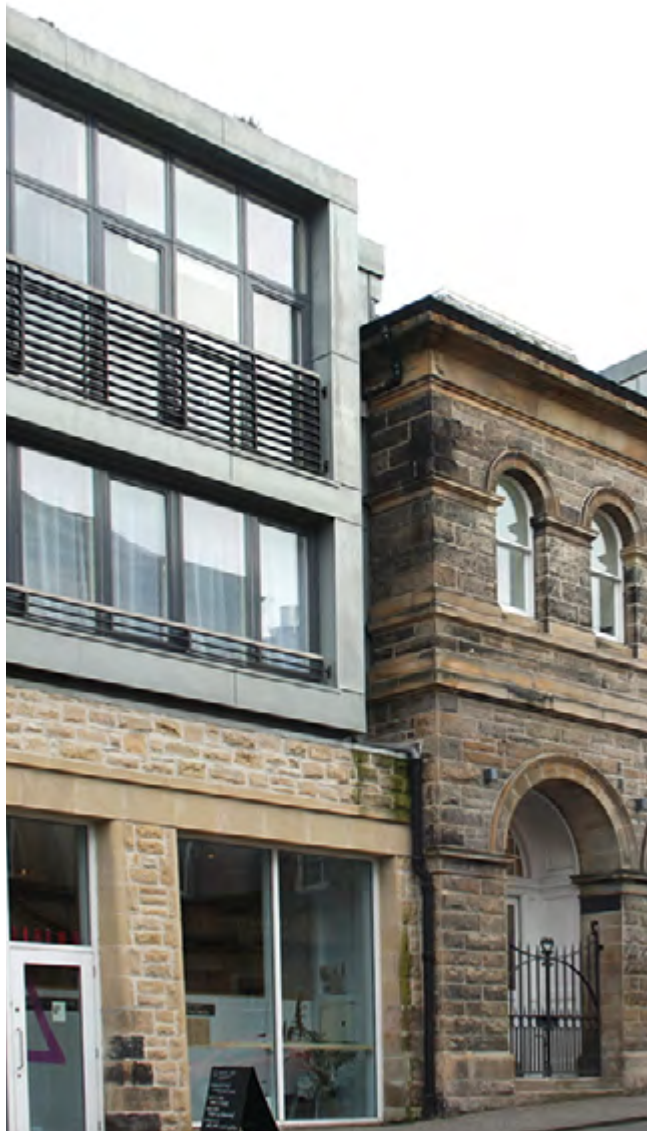
Using zinc to provide striking contrast: Infirmary St. - The zinc cladding combined with the modern building form for Dovecot Studio provides a positive contemporary contrast to the historic former Infirmary Street Baths building.
