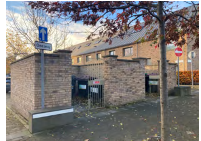
Accessible bin enclosures, Leith Fort - These carefully designed bin stores are discrete but easily accessible
