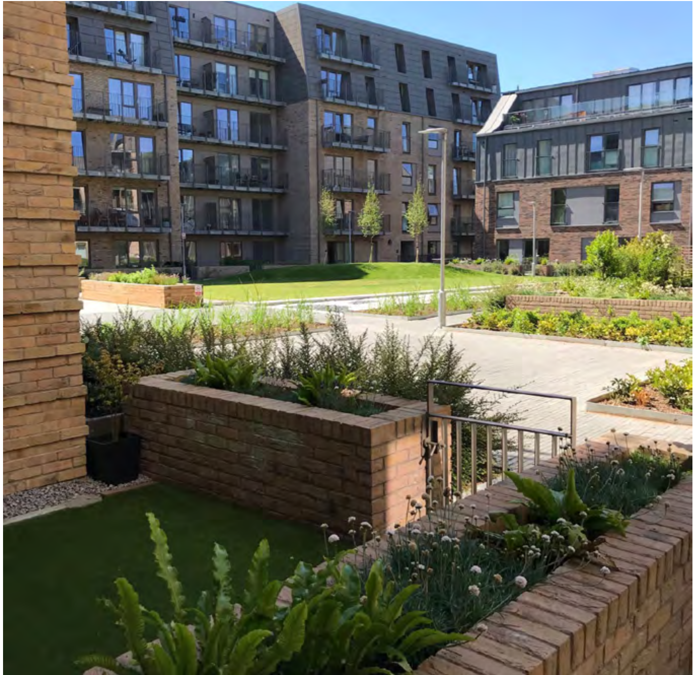
Providing high density homes with quality green space - At this relatively high density development at Canonmills Gardens, residential amenity is supported through a mix private gardens, balconies and communal open space.
