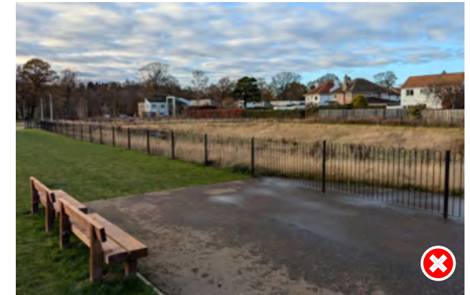
Limiting potential benefits through fencing - This SuDS basin limits the opportunities to maximise amenity and biodiversity benefits by being fenced off from the surroundings. This type of SuDS solution does not conform with the guidance recommended in this chapter. In general, carefully designed SuDS solutions avoid the need for fencing.
