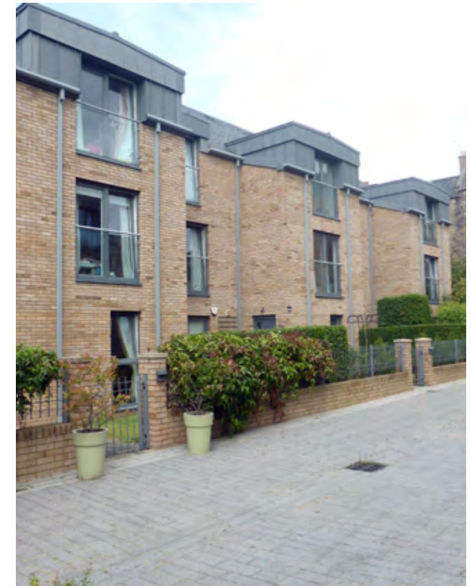
Incorporating family housing - The inclusion of townhouses in this development on McDonald Place provides a good option for families.
