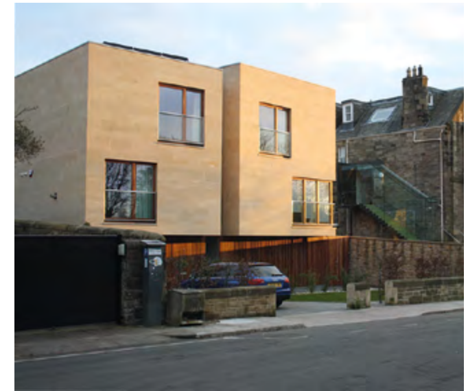
Modern development with a similar scale, Wester Coates Gardens - This villa has large windows which help to integrate it with the scale of surrounding historic villas. The proportions of stonework help also.
