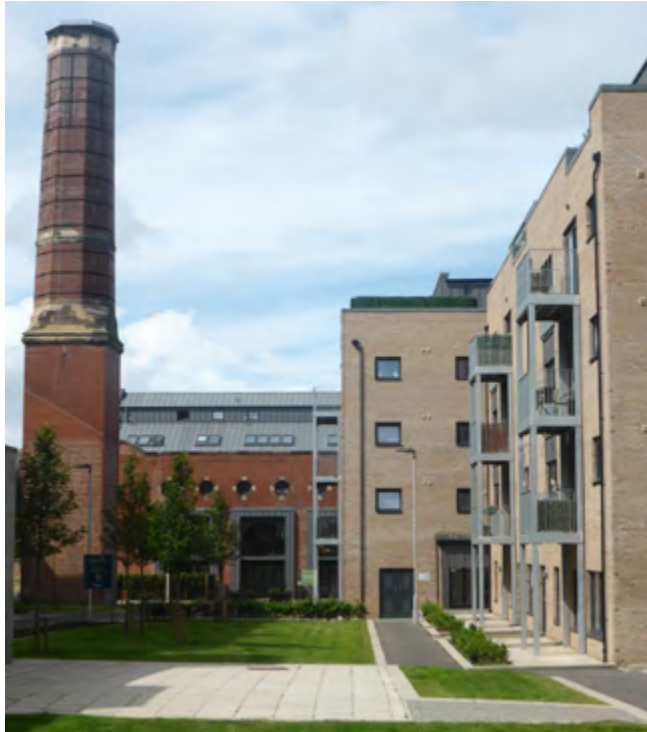
Retention of existing buildings - As part of the redevelopment of the former engine yards at Shrubhill, the conversion of the redundant tram sheds has safeguarded an important landmark that makes a special contribution to the surrounding area, while retaining the embodied carbon of the buildings.
