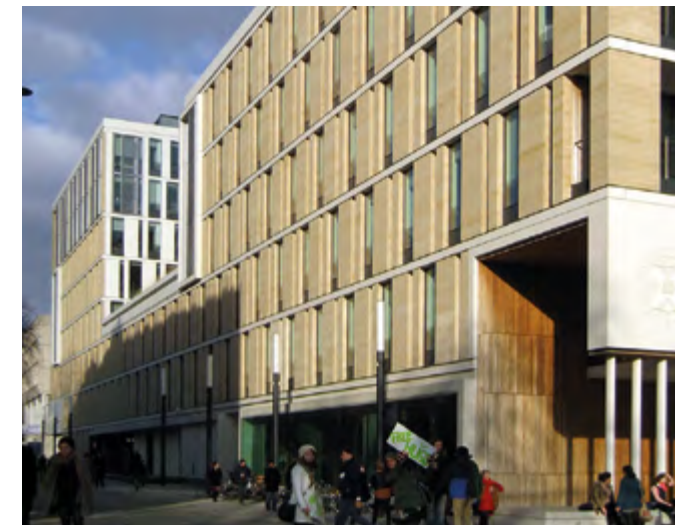
Informatics Forum: Charles Street - Sandstone is built into vertically proportioned panels which are used to order the design of the elevations.
