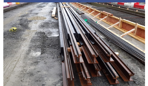
Delivery of rail to Leith Walk
