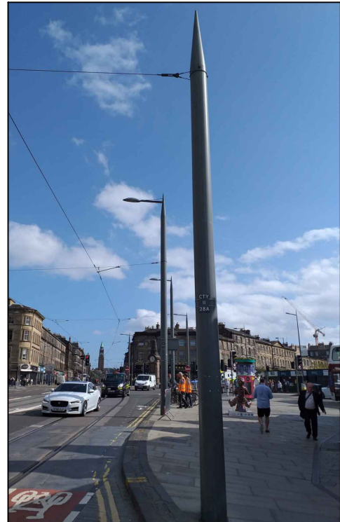
TYPICAL OLE POLE
